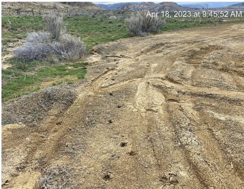
Sediment migration exiting location and vehicle tracking
