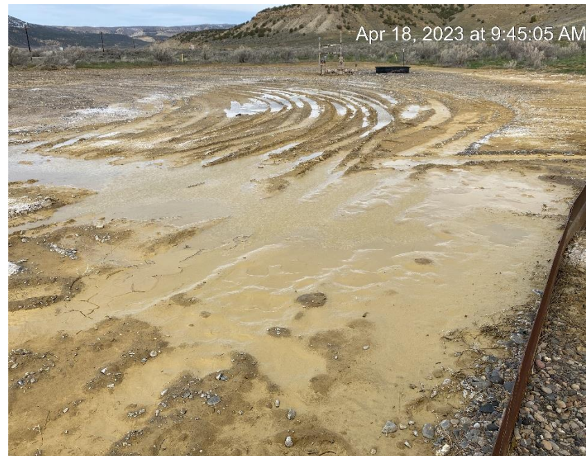
Lack of stabilization and vehicle tracking
