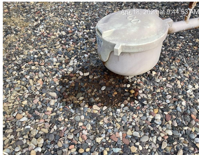
Crude oil loadline soil staining
