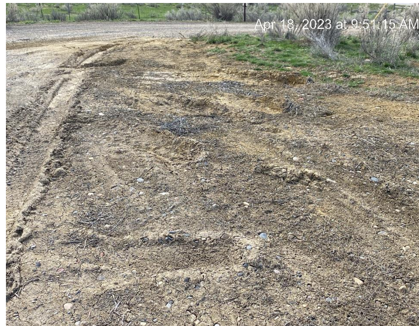
Sediment migration and vehicle tracking leaving location
