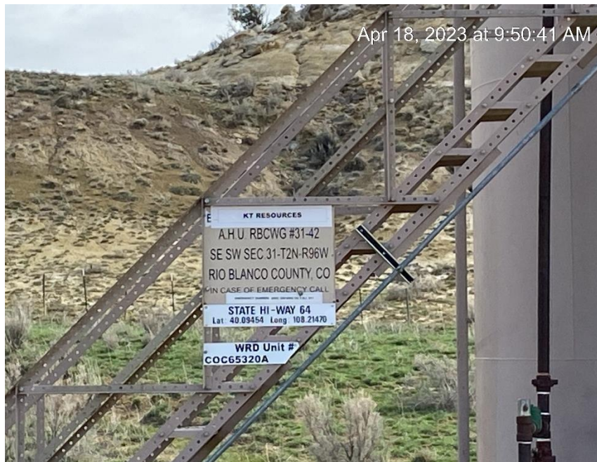
Tank sign missing well API Number
