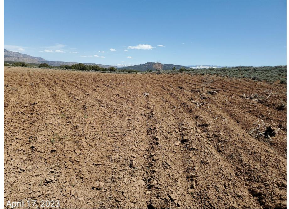
**Photo 1:** Photos taken from the west end of the Location, facing northeast and southeast. Photos shows Location has been recontoured, soils replaced, and decompacted.
