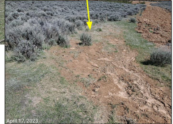
**Photo 10:** Stormwater and erosion control BMPs at the access road remain missing or insufficient. Photos right show sediment transport/deposition on undisturbed adjacent areas.
