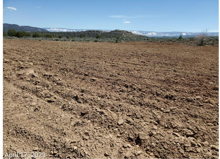
**Photo 2:** Photos taken from the north end of the Location. Photos 2-3 provide an overview of the Location from east, southeast, southwest to west. Photos show Location has been recontoured, soils replaced, and decompacted. Photos also show stormwater and erosion control BMPs, and BMPs to stabilize the soils remain missing or insufficient; soils left exposed and at risk to wind and water erosion; surface roughening alone inadequate.
