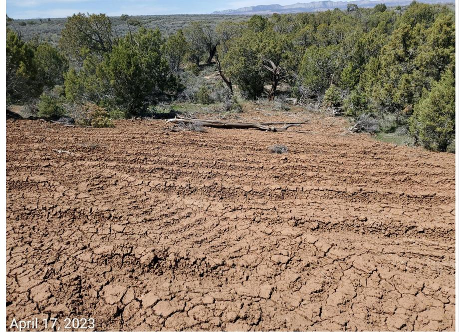
**Photo 7:** Photos taken from the Location. Photos examples showing stormwater and erosion control BMPs remain missing or insufficient; soils have been left exposed, unstabilized and at risk to wind/water erosion. BMPs to manage runoff and minimize off-site sediment transport along the perimeter also missing or insufficient; surface roughening alone inadequate.
