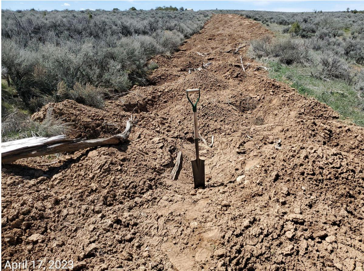
**Photo 8:** Photo taken from the access road. Photo shows Operator has re “pot-holed” the access road, resulting in large holes and soil piles; soils have been left unstabilized; access road has not been properly contoured and stabilized; seeding activities at access road not apparent.
