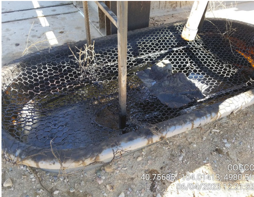
Photo 7 – Oily Waste at Pumping Unit
