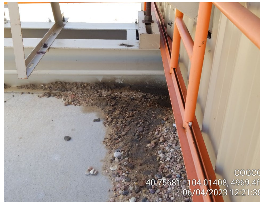
Photo 6 – Stained Soil at Gas Engine
