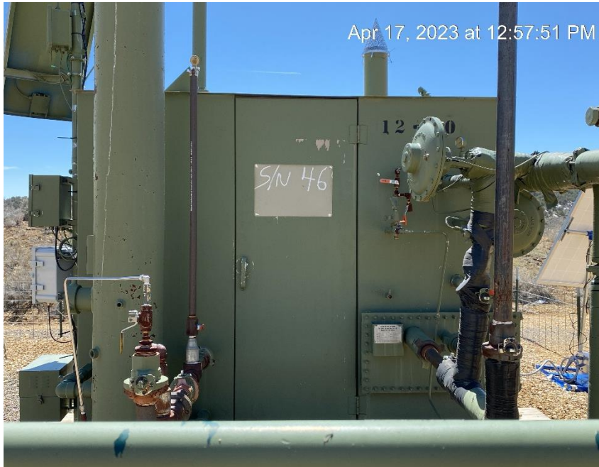
No gas meter calibration card visibly displayed
