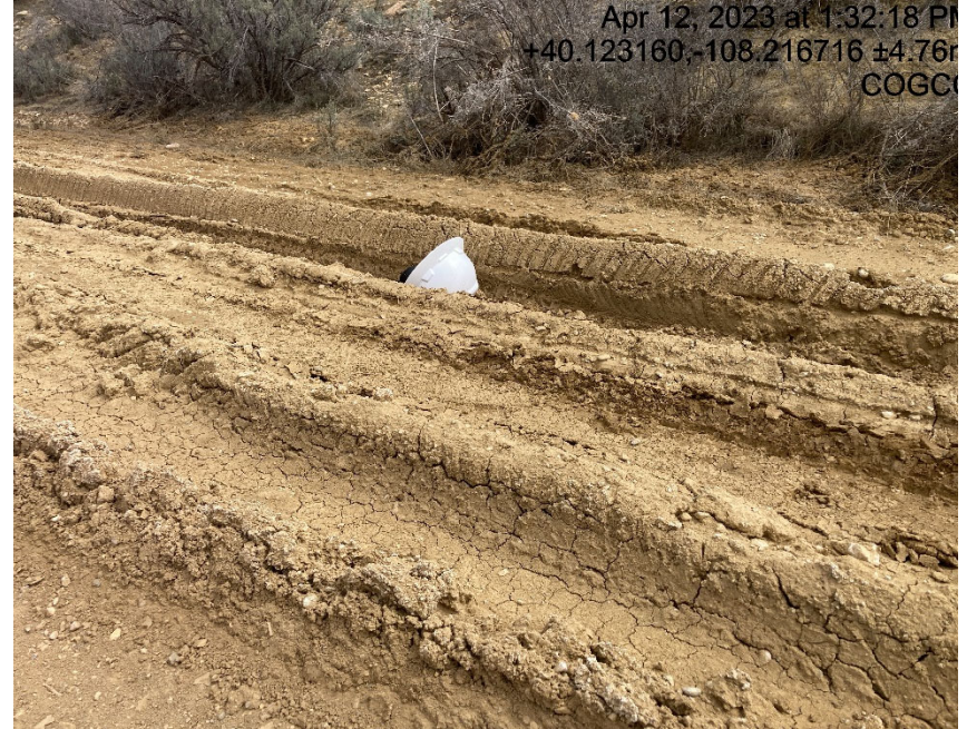
Lack of stabilization/compaction and failing BMP's
