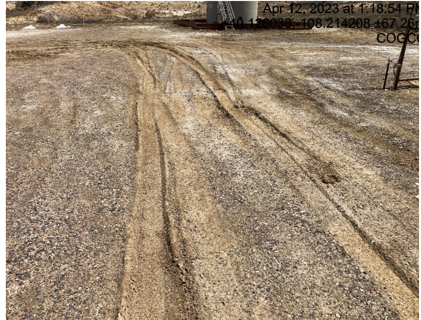
Lack of stabilization/compaction and failing BMP's
