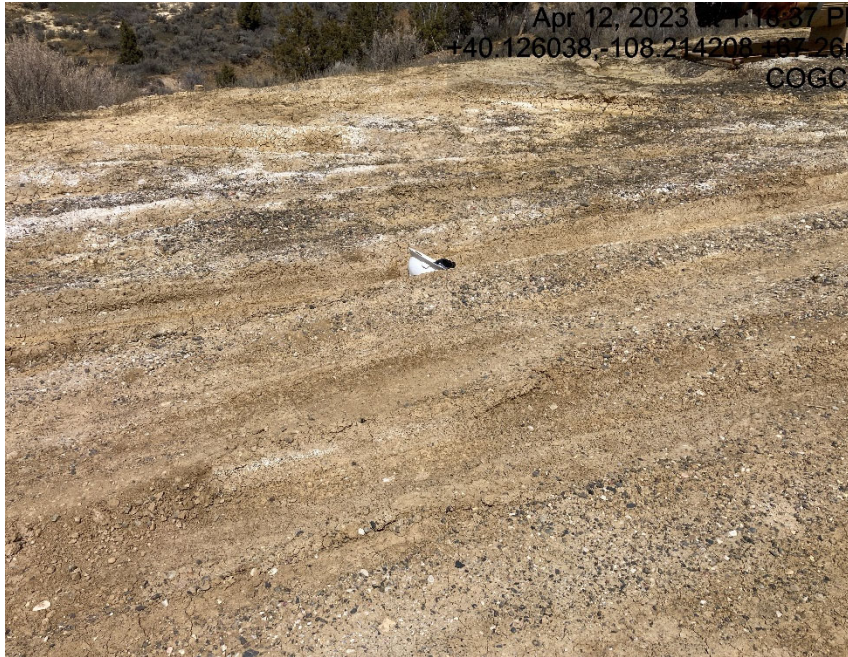
Lack of stabilization/compaction and failing BMP's
