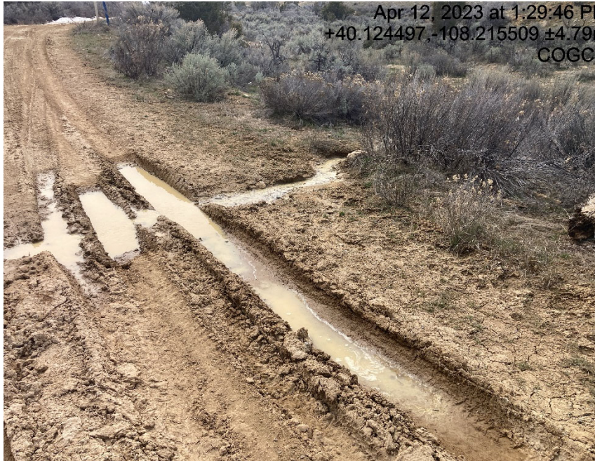
Lack of stabilization/compaction and failing BMP's
