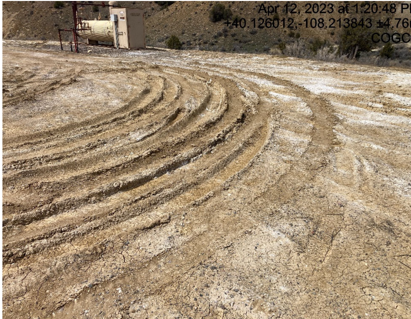
Lack of stabilization/compaction and failing BMP's
