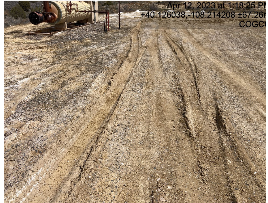
Lack of stabilization/compaction and failing BMP's
