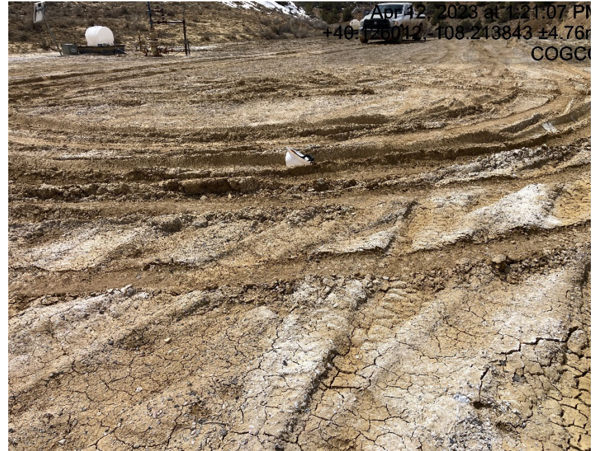
Lack of stabilization/compaction and failing BMP's
