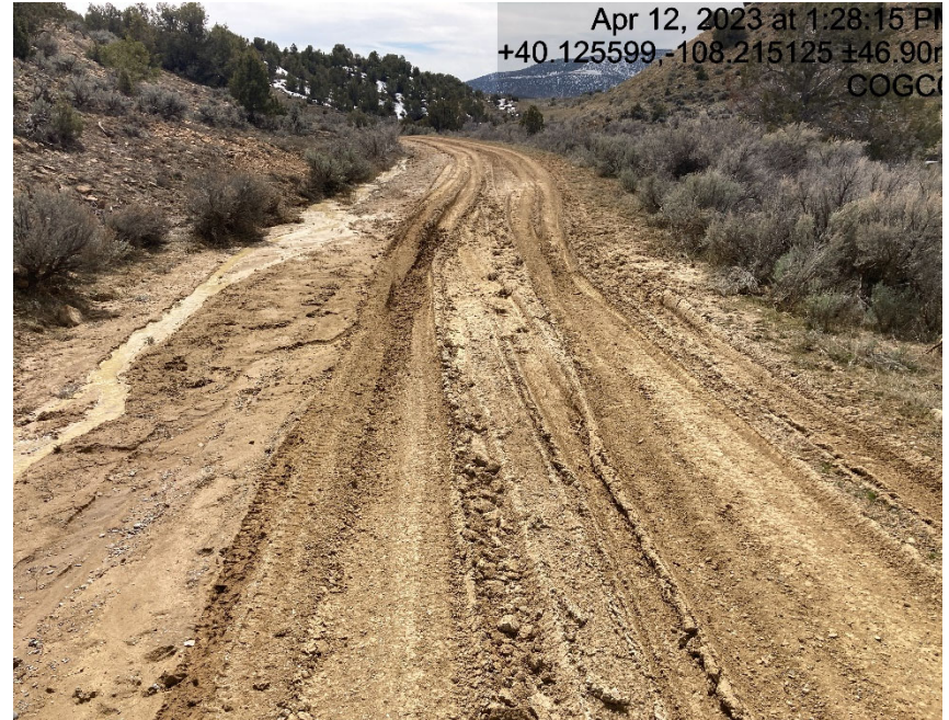
Lack of stabilization/compaction and failing BMP's
