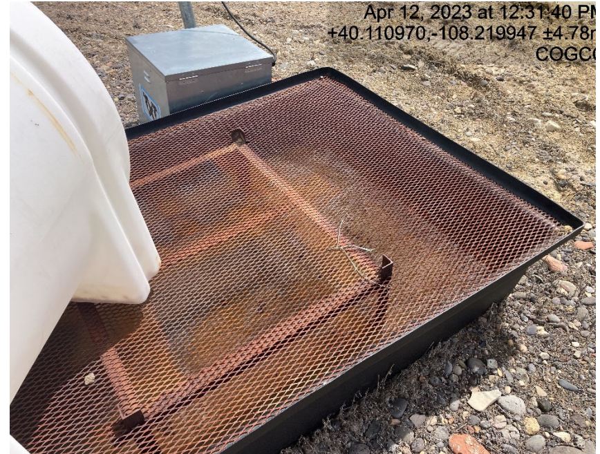
Chemical containment is full of fluid and unused/stored equipment
