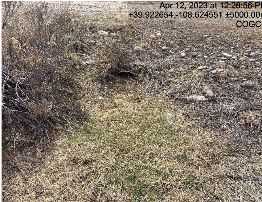
Entrance to location culvert outlet failing
