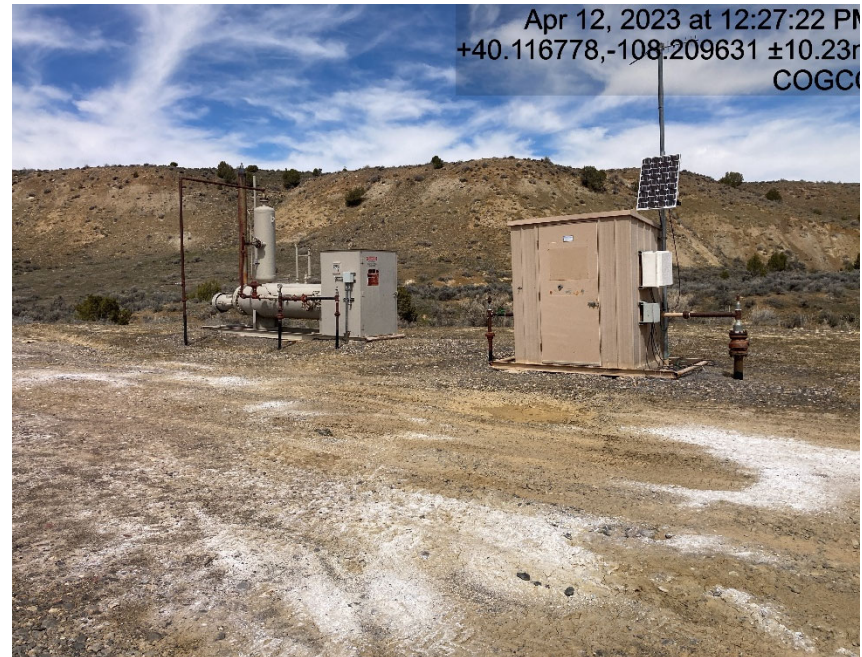
Separator and meter house
