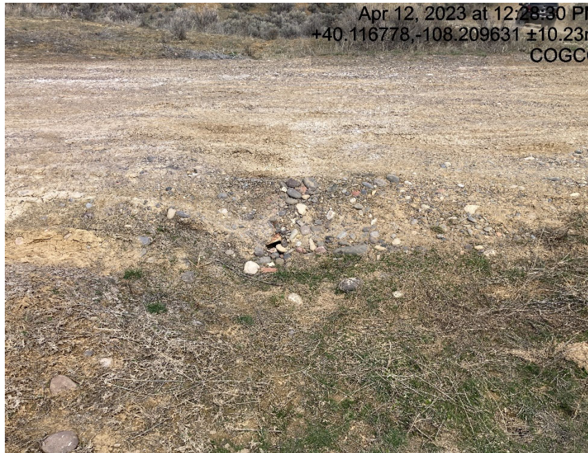
Entrance to location culvert inlet failing
