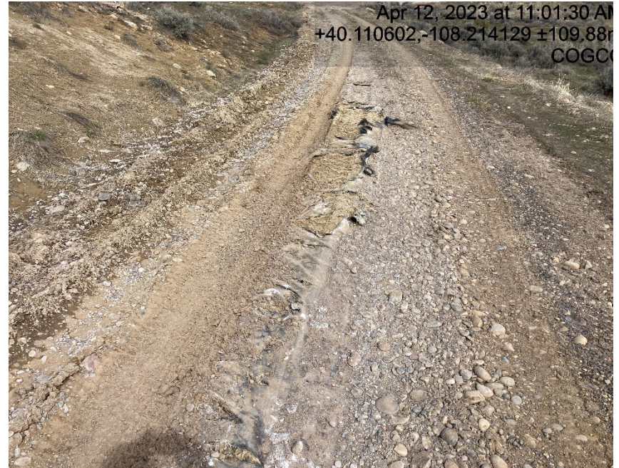
Access road lack of stabilization
