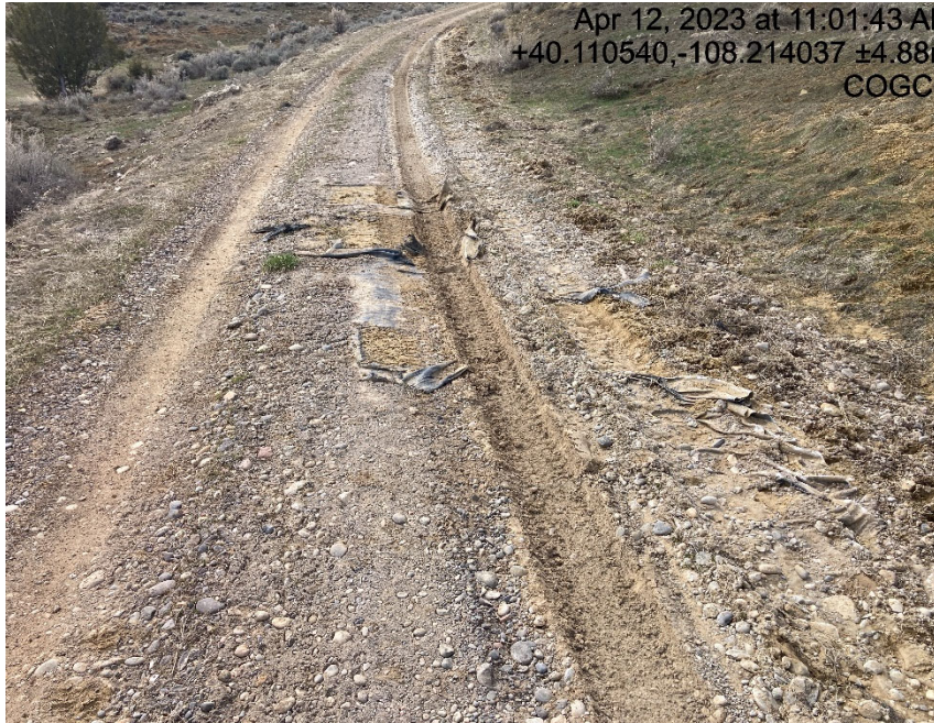
Access road lack of stabilization
