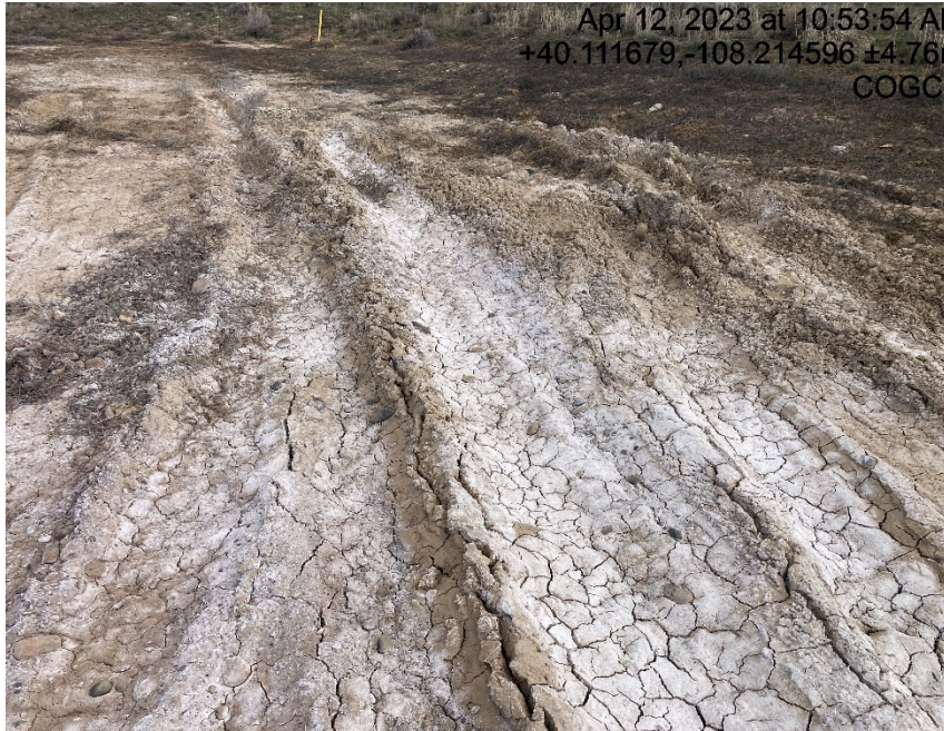
Lack of stabilization/compaction
