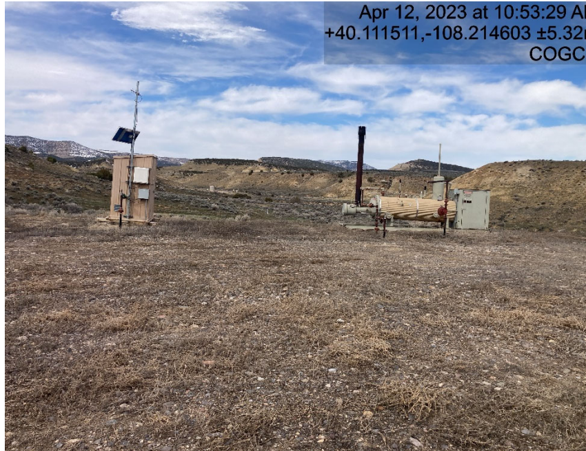
Horizontal separator and meter house
