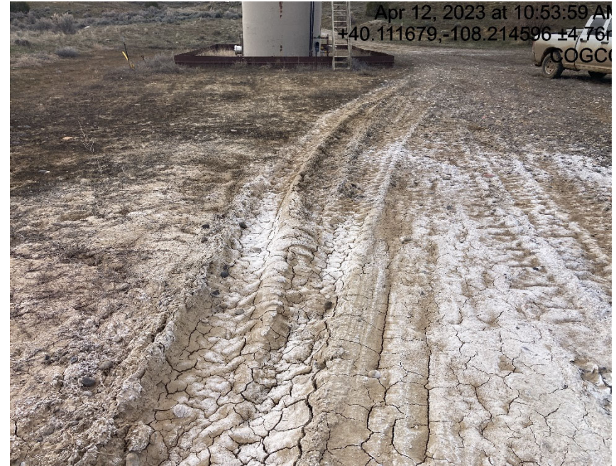
Lack of stabilization/compaction
