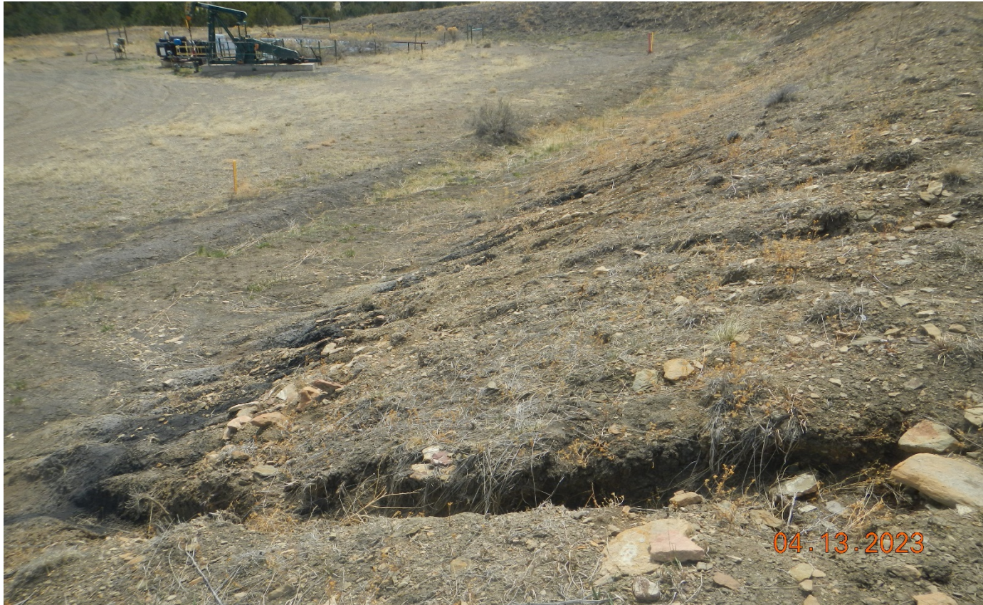
Photo 4. There is an erosion channel along the cut slope that needs to be repaired and stabilized.
