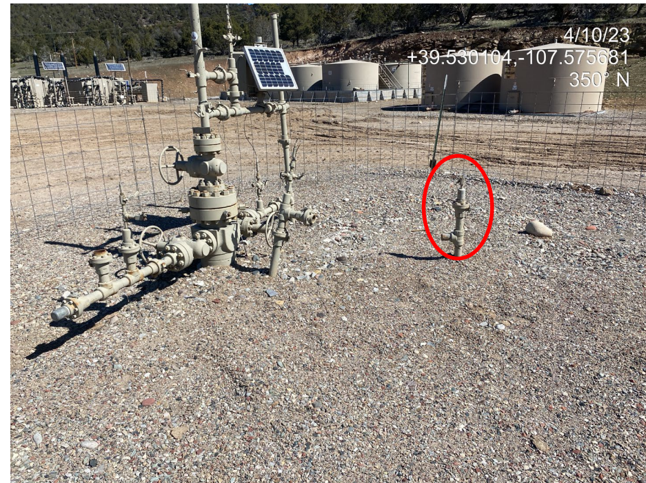
Photo 1. Photos show a flowline riser remaining at plugged and abandoned well 045-17865. OOSLAT not applied.
