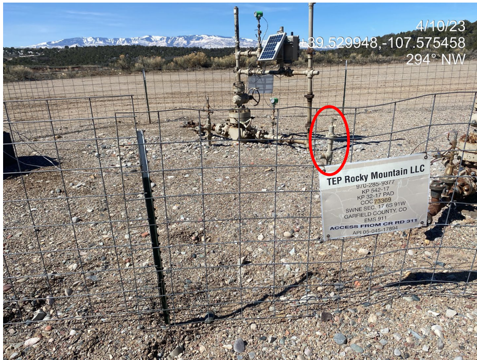
Photo 2. Photos show a flowline riser remaining at plugged and abandoned well 045-17894. OOSLAT not applied.
