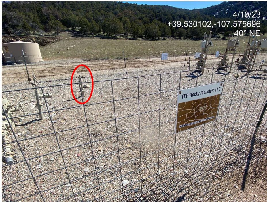
Photo 1. Photos show a flowline riser remaining at plugged and abandoned well 045-17865. OOSLAT not applied.
