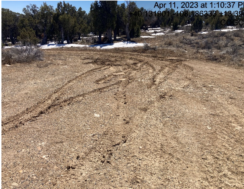
Lack of stabilization/compaction
