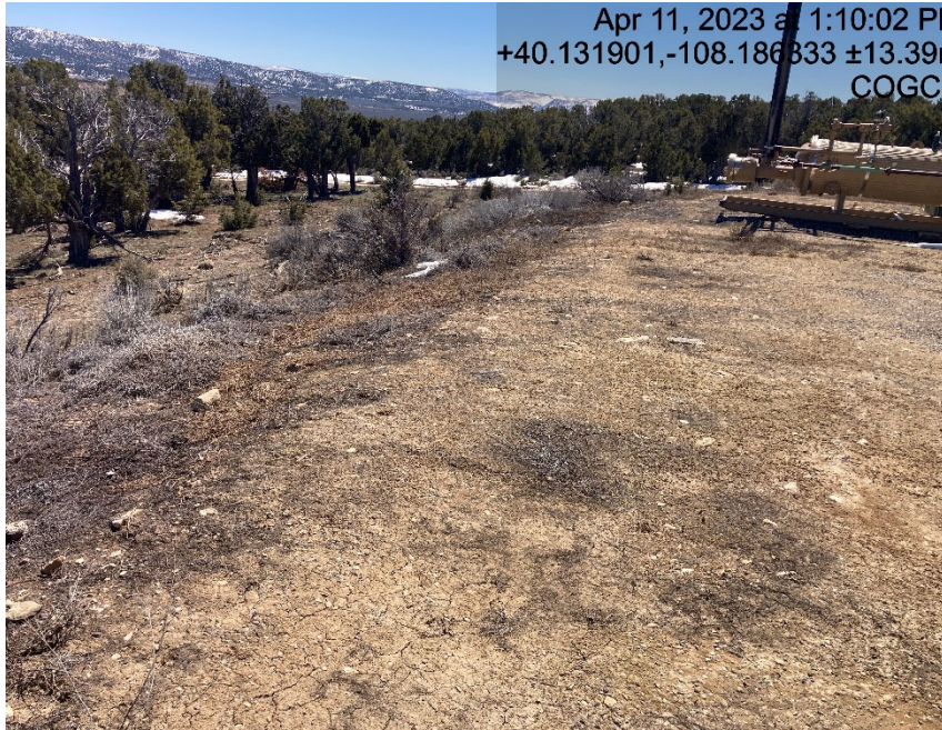
Lack of BMP's to prevent sediment migration from location
