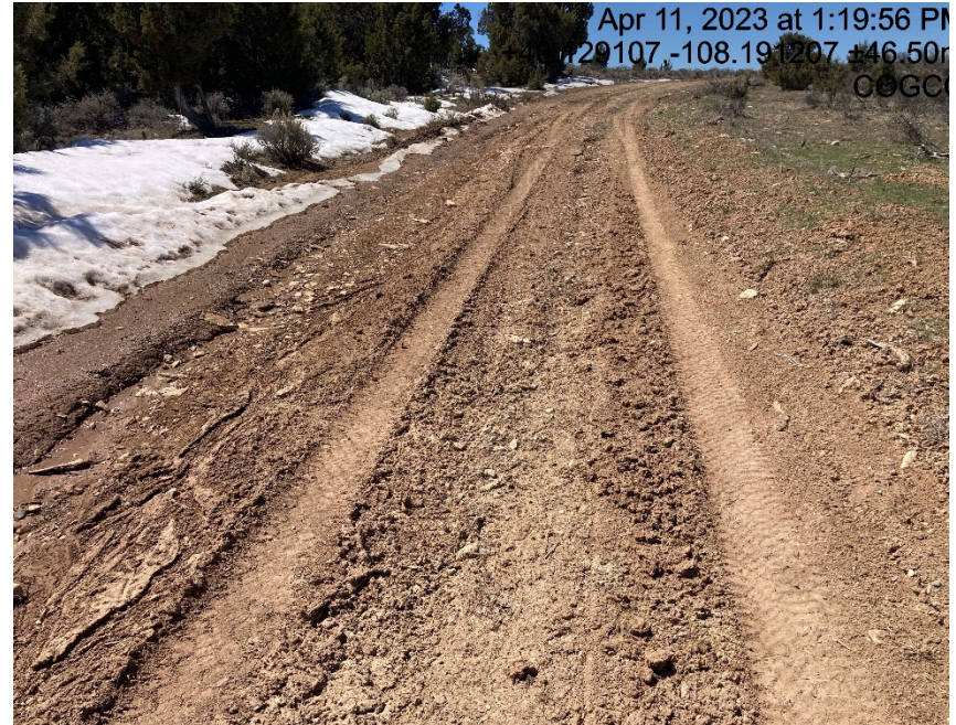
Access road erosion/ lack of stabilization
