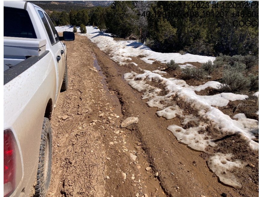
Access road erosion/ lack of stabilization
