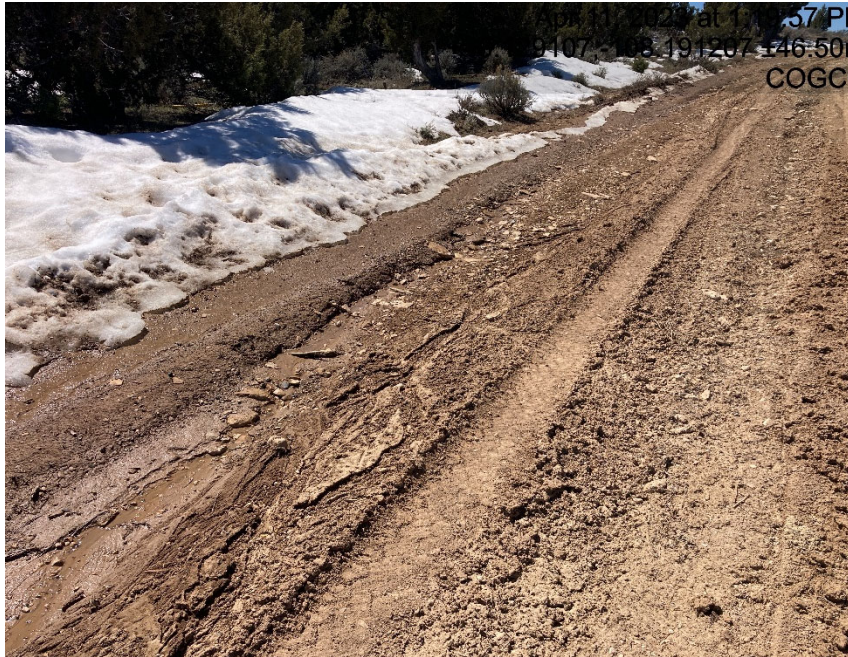
Access road erosion/ lack of stabilization
