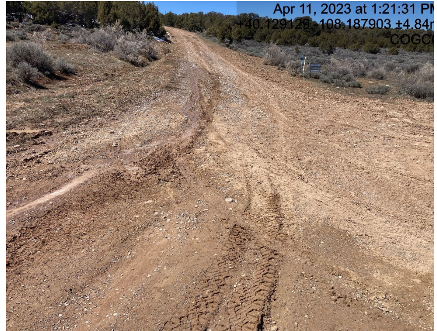
Access road erosion/ lack of stabilization
