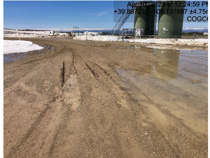
Lack of stabilization/compaction
