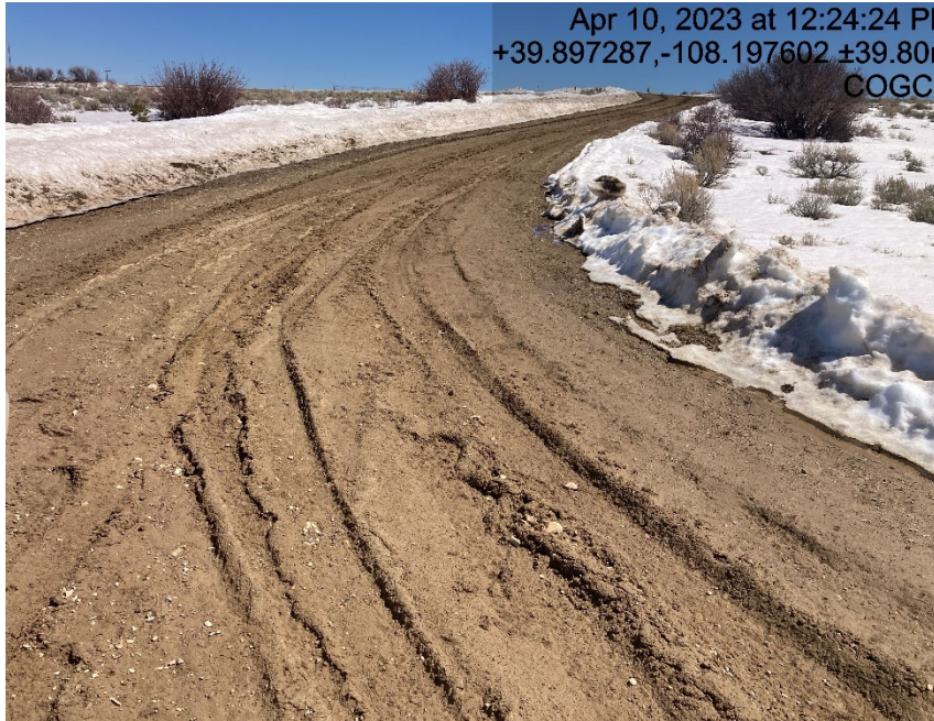
Lack of stabilization/compaction
