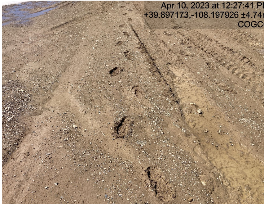
Lack of stabilization/compaction
