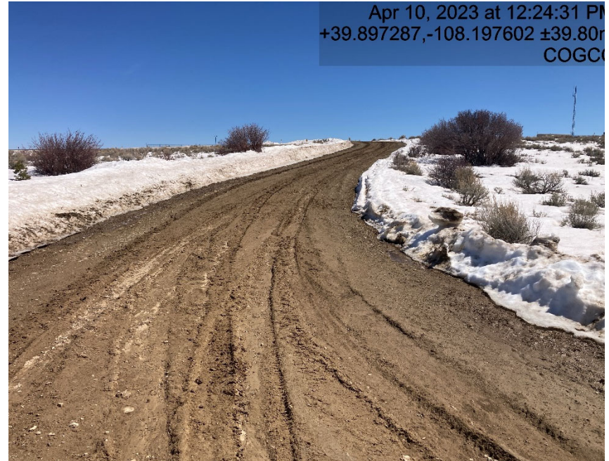
Lack of stabilization/compaction
