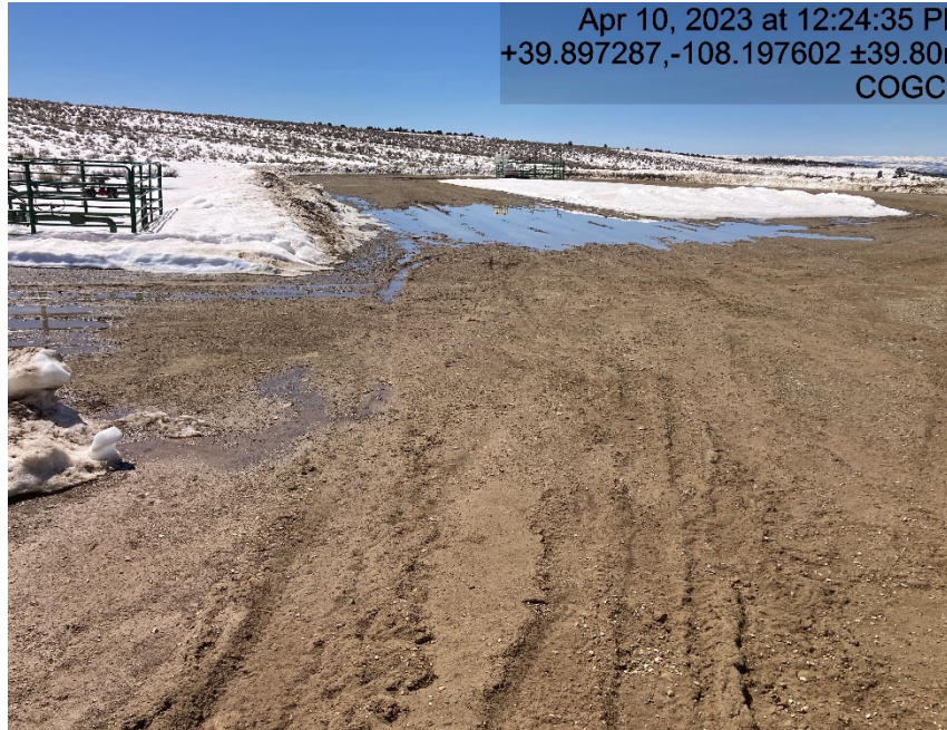
Lack of stabilization/compaction
