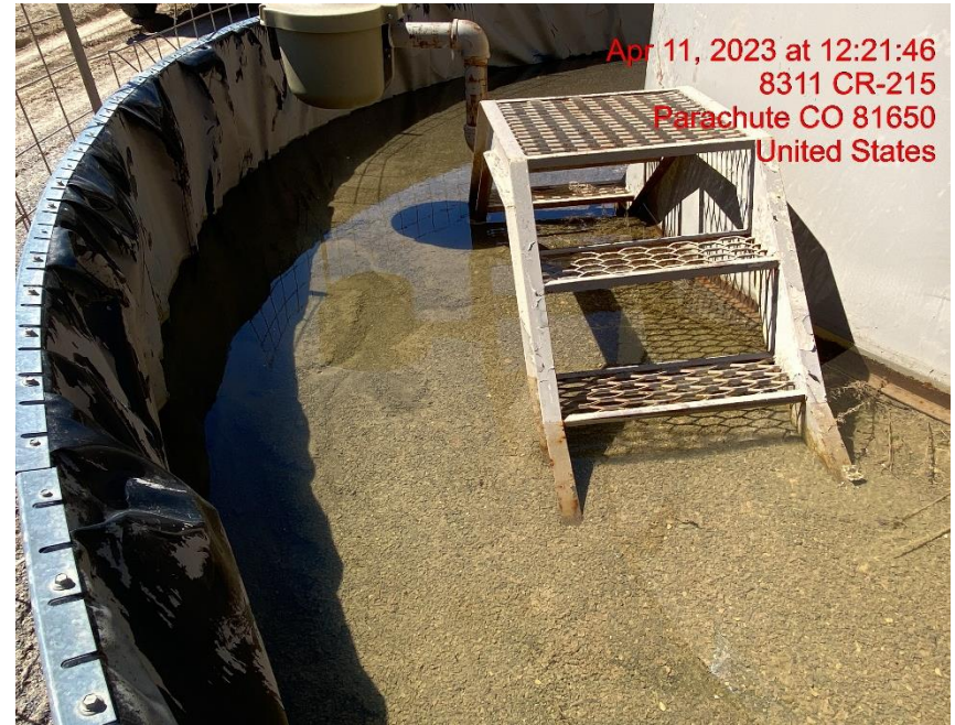
Inadequate Berm Capacity – Photo #02122
