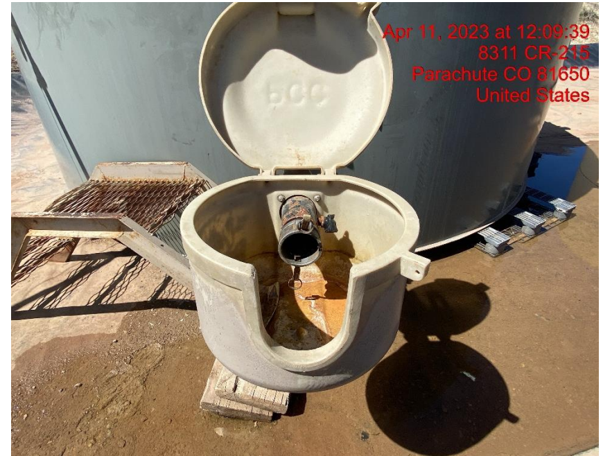
Open-Ended Load Line – Photo #02109
