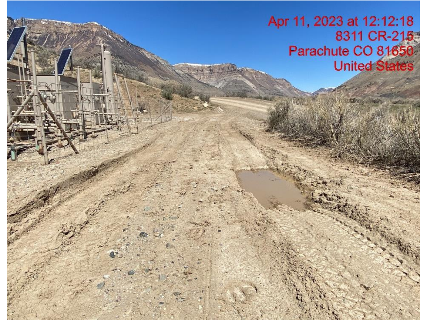
Inadequate Vehicle Tracking BMP – Photo #02115
