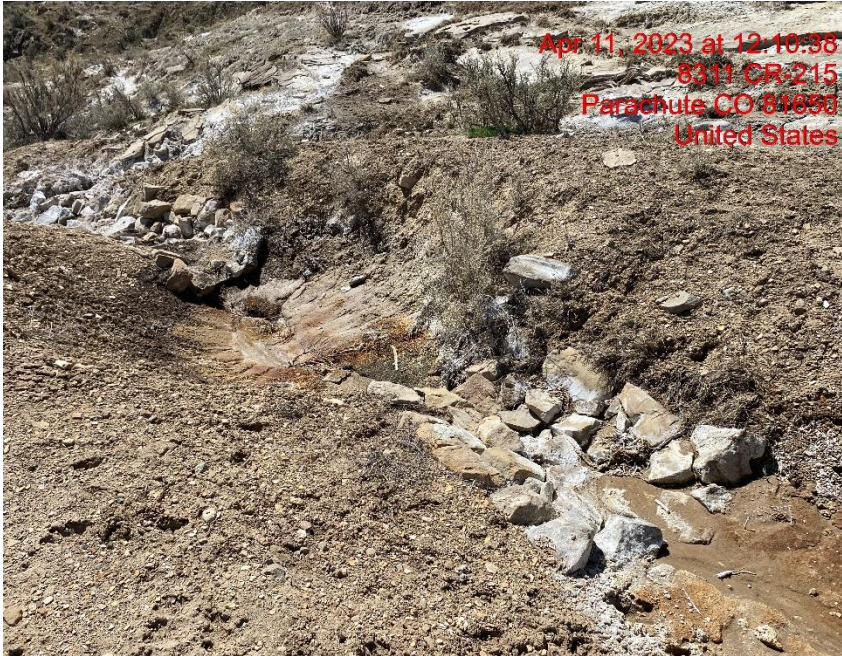
Check Dam Sediment Build-Up – Photo #02112
