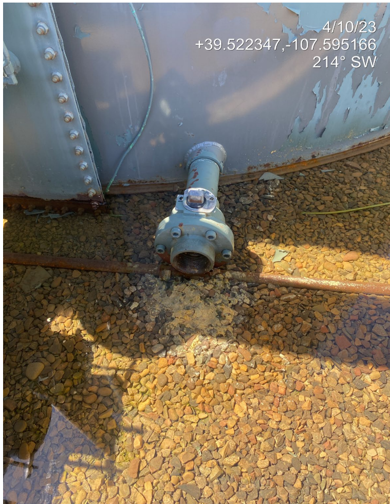
Photo 4. Photos show drain lines without bull plugs and staining below the lines.
