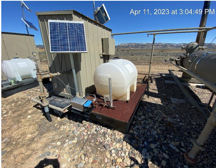
Chemical tank labels missing and/or illegible
