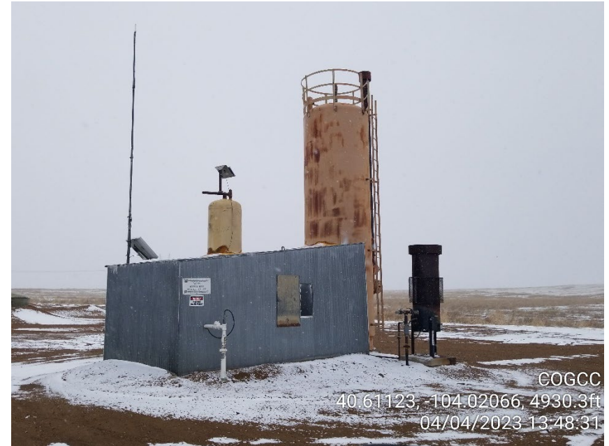
Photo 2 – Heater Treater and ECD
