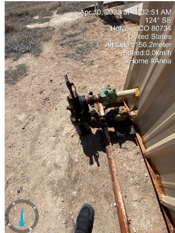
6. Gas blowing at 2" T before going into ground, also leaking on same line inside shed.
