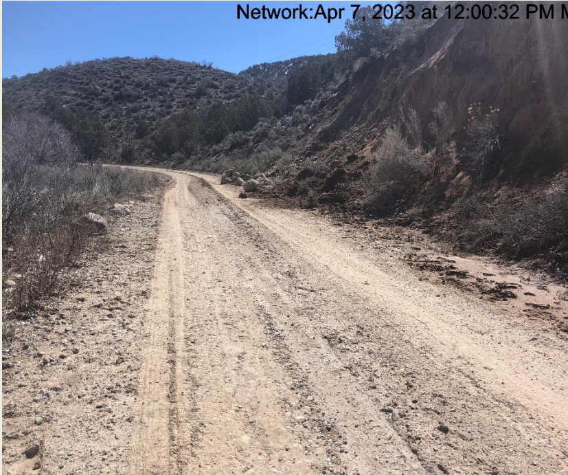
Photo #9606 Access road cut slope lacks stabilization.
