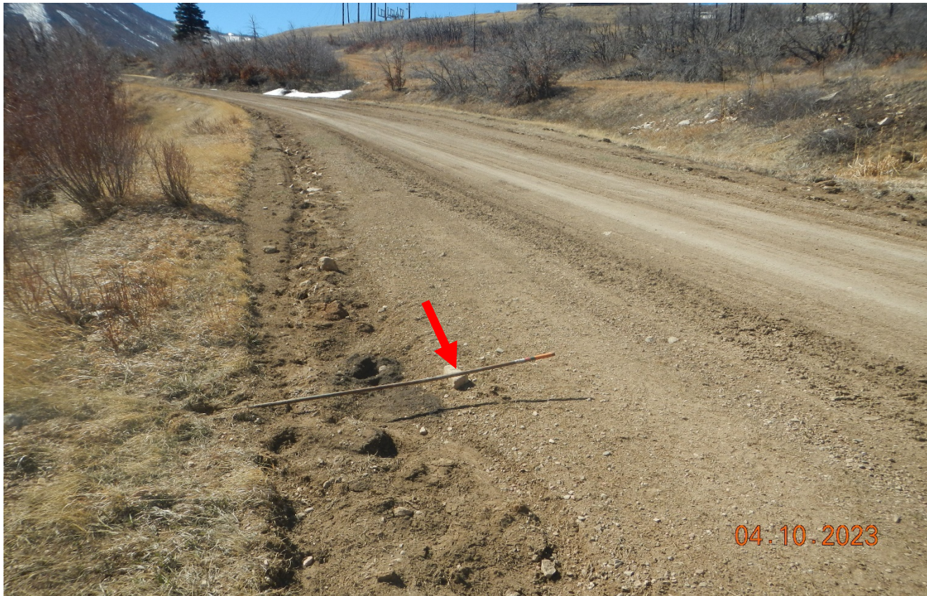
Photo 2. Facing southeast ascending the hill toward the location. There has been grading performed which has widened the road and pulled up the metal rebar which needs to be removed or repaired and made more visible.
