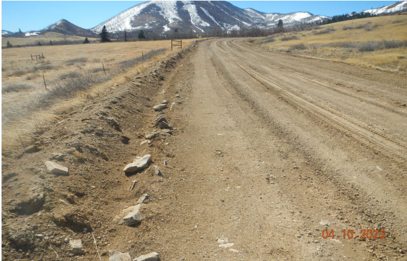
Photo 4. Facing southeast ascending the hill toward the location. Grading has pushed out material into a berm which is creating more of a disturbance and not allowing stormwater to be diverted off the road. There is a long stretch of the road where stormwater will be directed down the road which will cause erosion.
