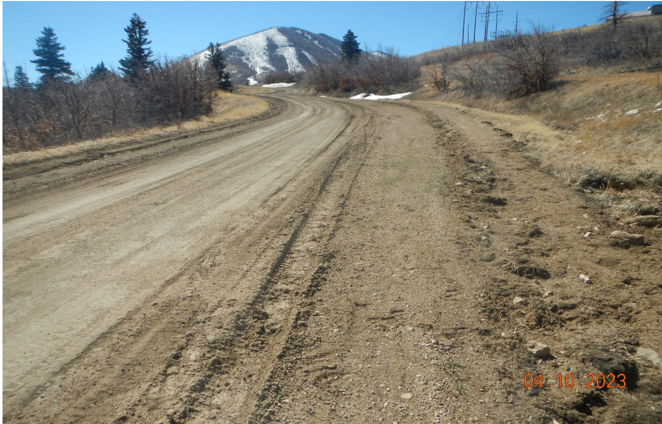
Photo 3. Facing southeast ascending the hill toward the location. The road has been widened along this area which will create more stormwater impact. Disturbance area of the road should be minimized.
