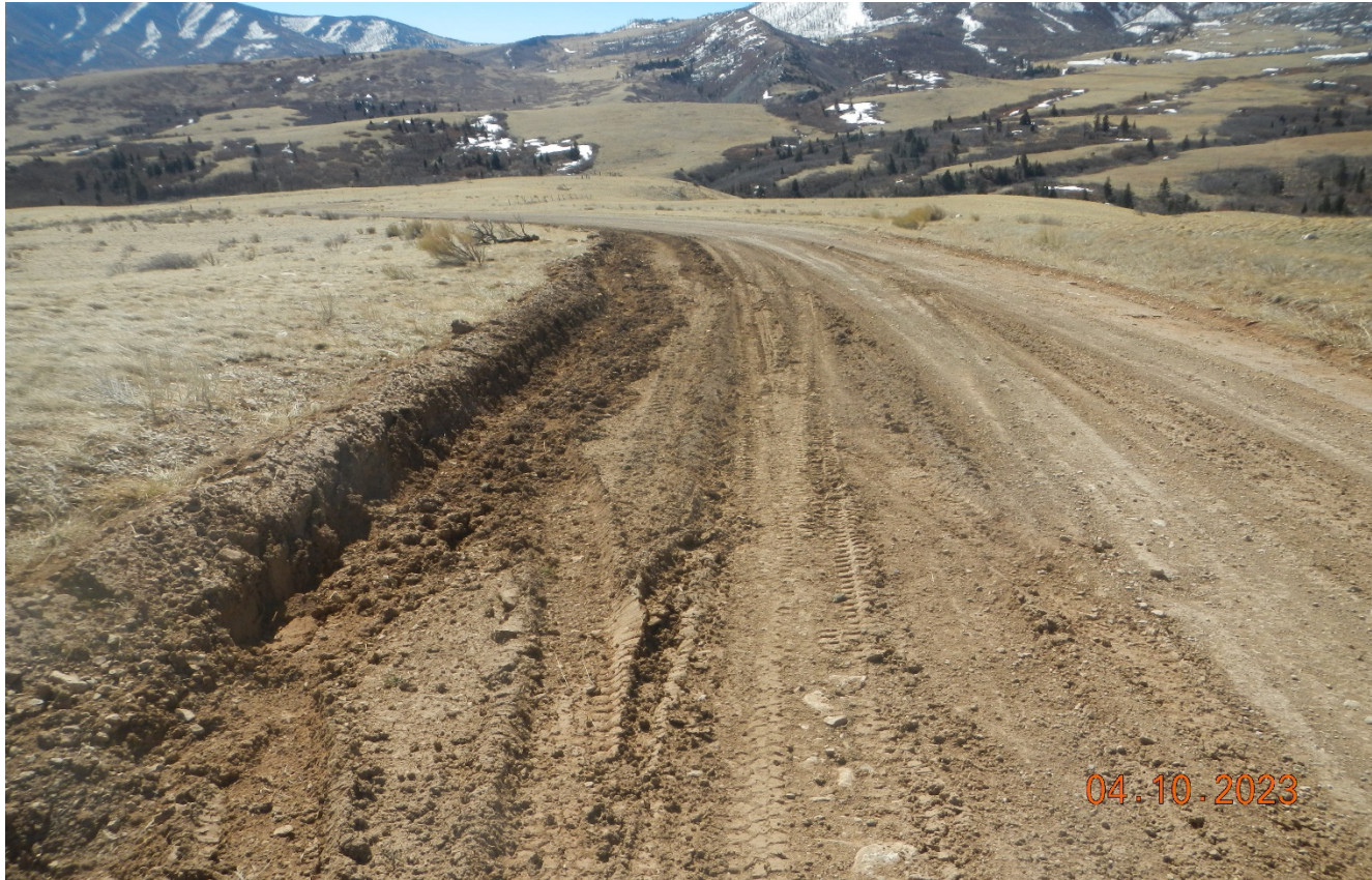
Photo 1. Facing south along the main road. It appears a vehicle slid off the road causing rutting disturbance that will need to be repaired.
