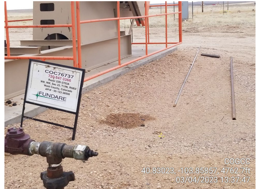
Photo 10 – 2703A Wellhead Sign – Stained Soil and Unused Pipe
