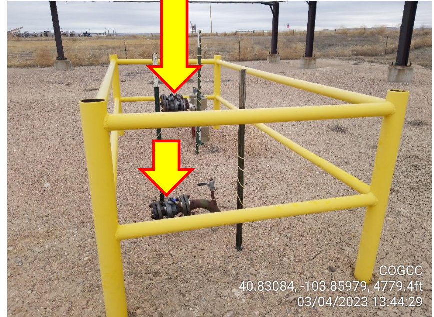
Photo 26 – Unmarked Risers
