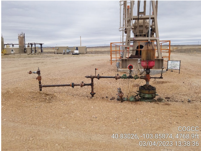
Photo 11 – 2712H Wellhead – Stained Soil
