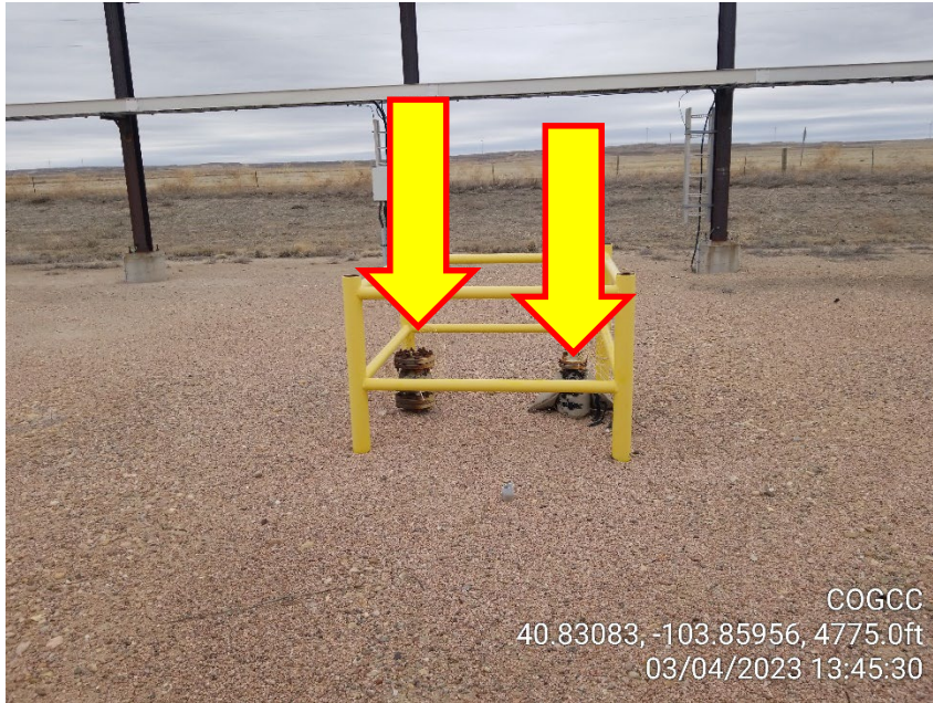
Photo 29 – Unmarked Risers
