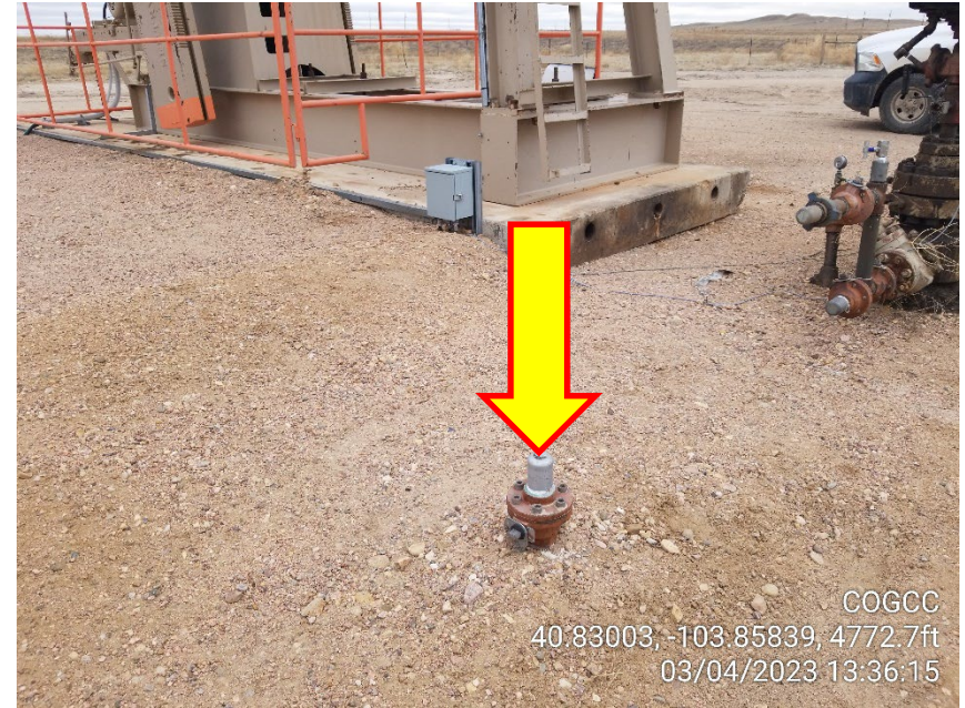
Photo 6 – Unmarked Riser
