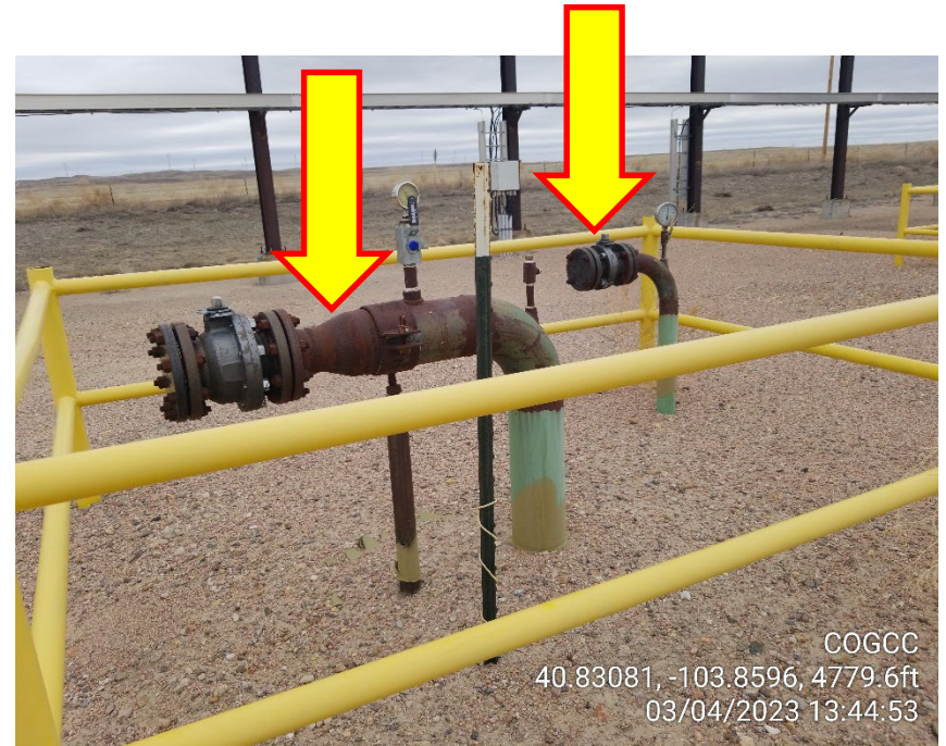
Photo 28 – Unmarked Risers
