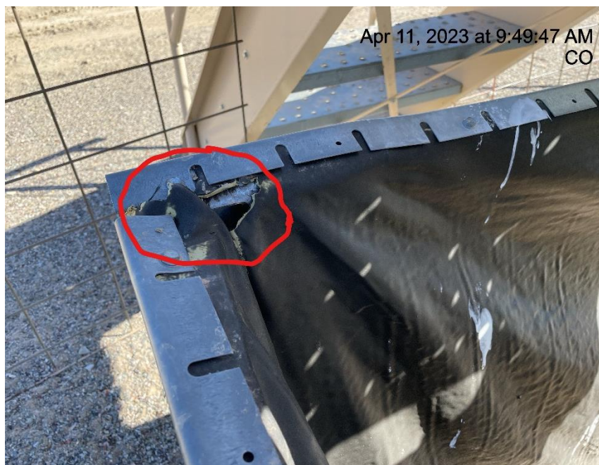
Photo # 4958 Containment liner needs maintenance
