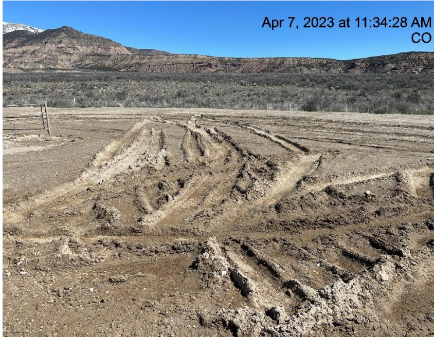
Photo # 4664 Lack of stabilization/compaction on location
