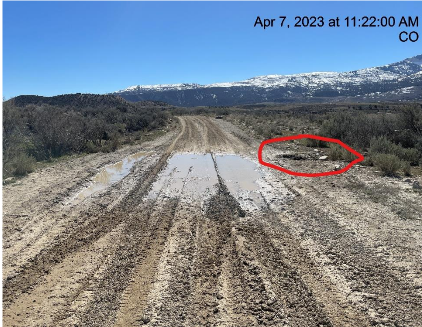
Photo # 4636 Erosion & transport of sediment off lease road/insufficient BMP's (approximately 1/10 th of a mile after the CLOUGH 111 pad)
