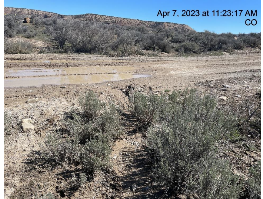
Photo # 4640 Erosion & transport of sediment off lease road/insufficient BMP's (approximately 1/10th of a mile after the CLOUGH 111 pad)
