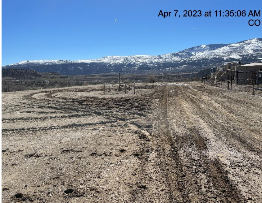
Photo # 4666 Lack of stabilization/compaction on location
