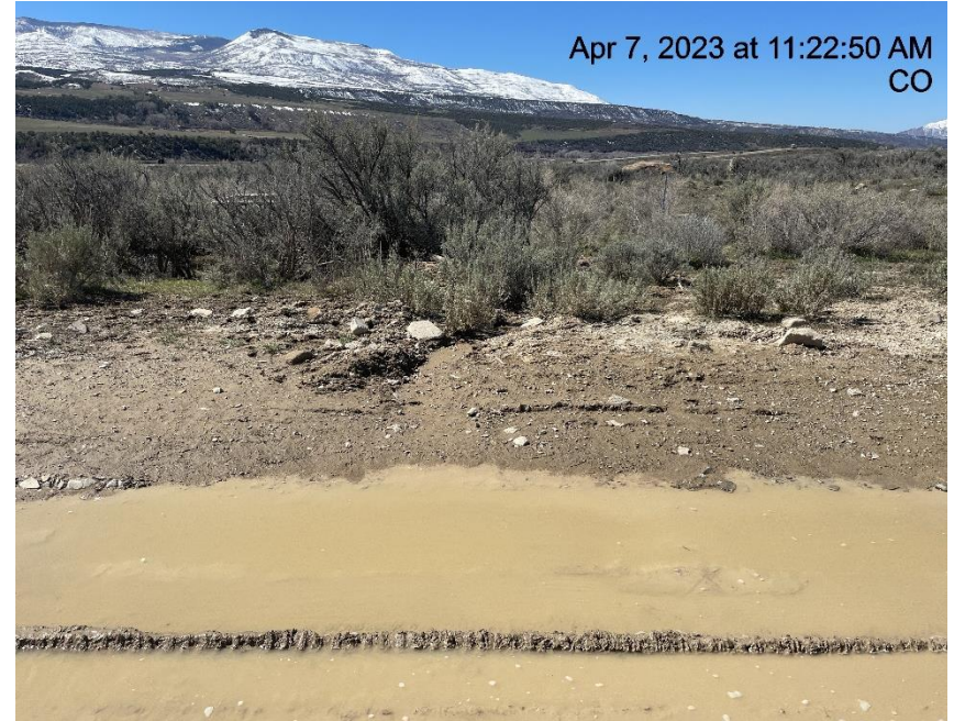
Photo # 4638 Erosion & transport of sediment off lease road/insufficient BMP's (approximately 1/10 th of a mile after the CLOUGH 111 pad)
