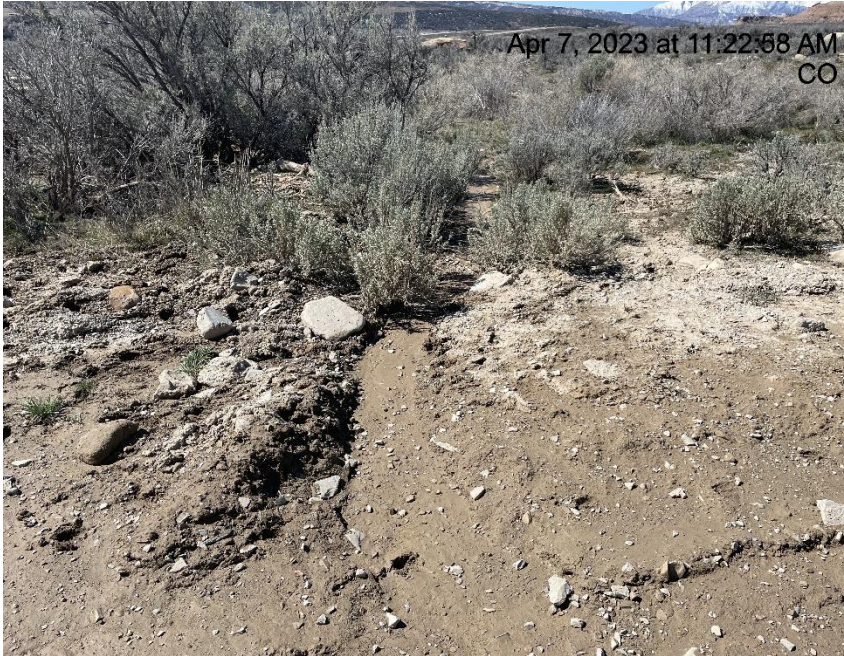
Photo # 4639 Erosion & transport of sediment off lease road/insufficient BMP's (approximately 1/10th of a mile after the CLOUGH 111 pad)
