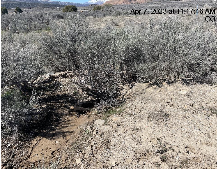
Photo # 4628 Erosion & transport of sediment off lease road/insufficient BMP's (approximately 2/10th of a mile after the CLOUGH 111 pad)
