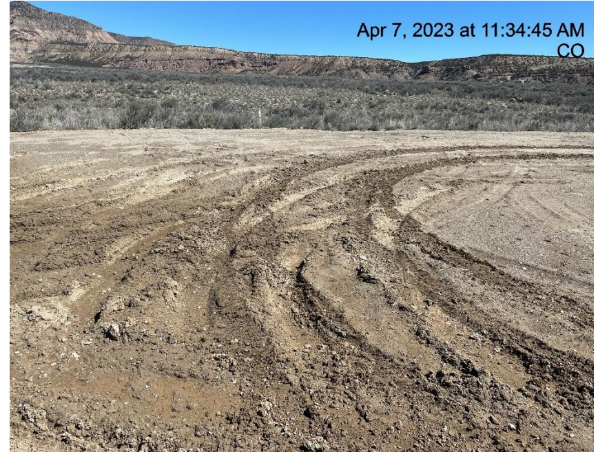
Photo # 4665 Lack of stabilization/compaction on location
