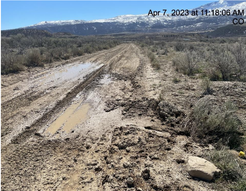
Photo # 4630 Erosion & transport of sediment off lease road/insufficient BMP's (approximately 2/10th of a mile after the CLOUGH 111 pad)
