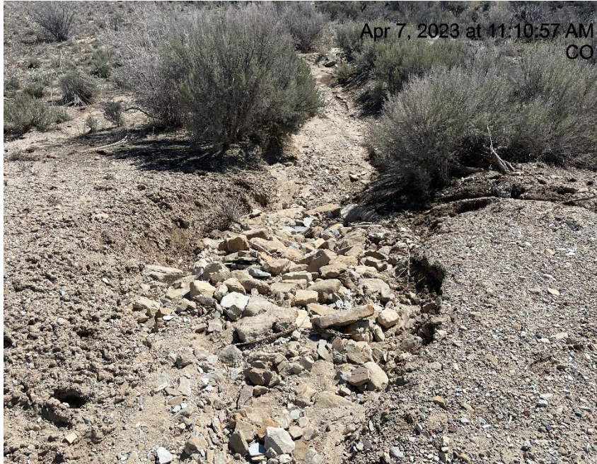
Photo # 4605 Rip Rap run needs maintenance (SE area of location)
