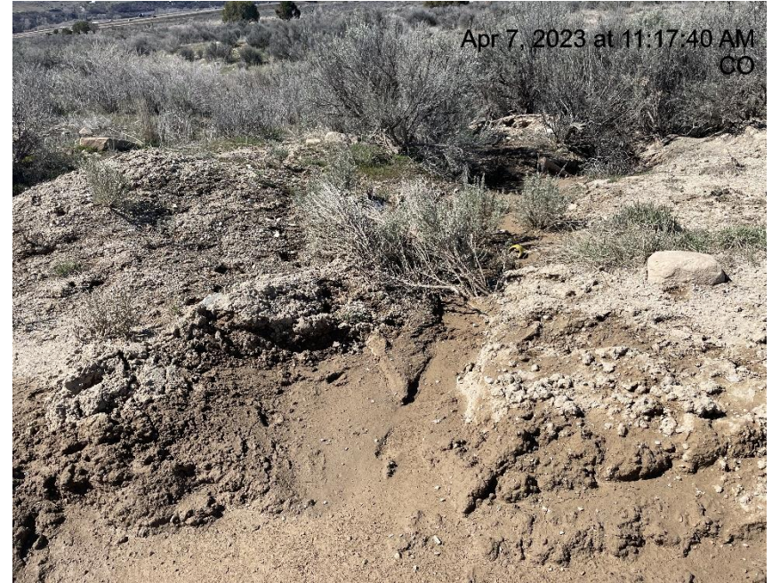
Photo # 4627 Erosion & transport of sediment off lease road/insufficient BMP's (approximately 2/10th of a mile after the CLOUGH 111 pad)
