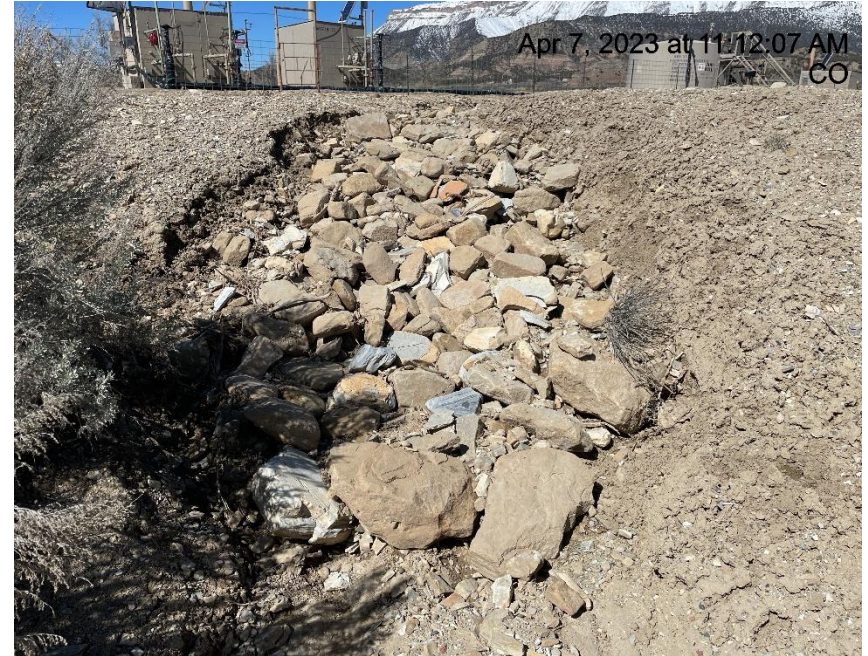
Photo # 4607 Rip Rap run needs maintenance (SE area of location)
