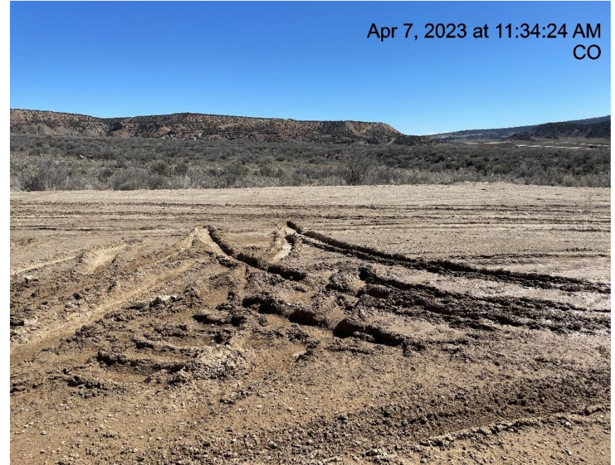
Photo # 4663 Lack of stabilization/compaction on location
