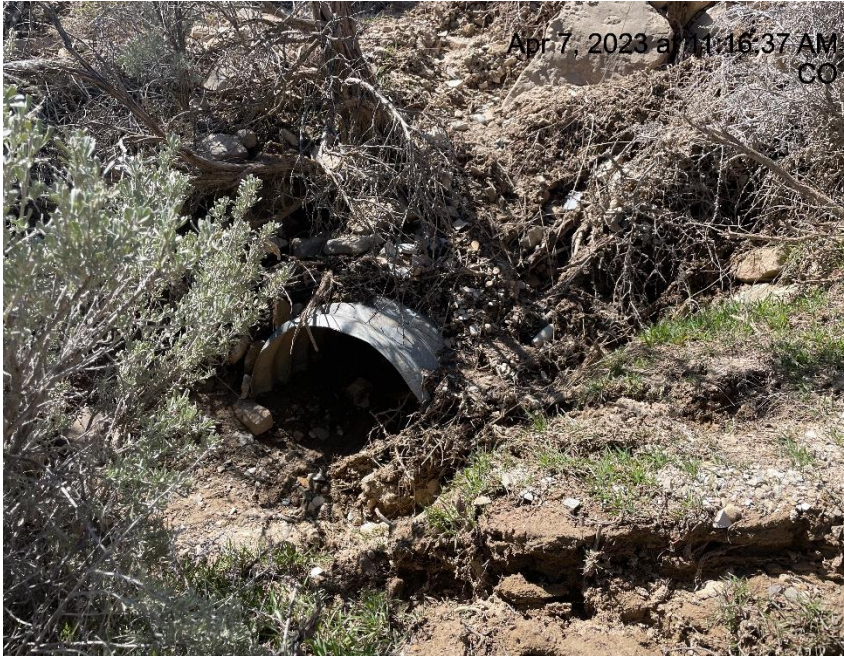
Photo # 4625 Culvert needs maintenance (on lease road 10-20 yards from entrance to location)
