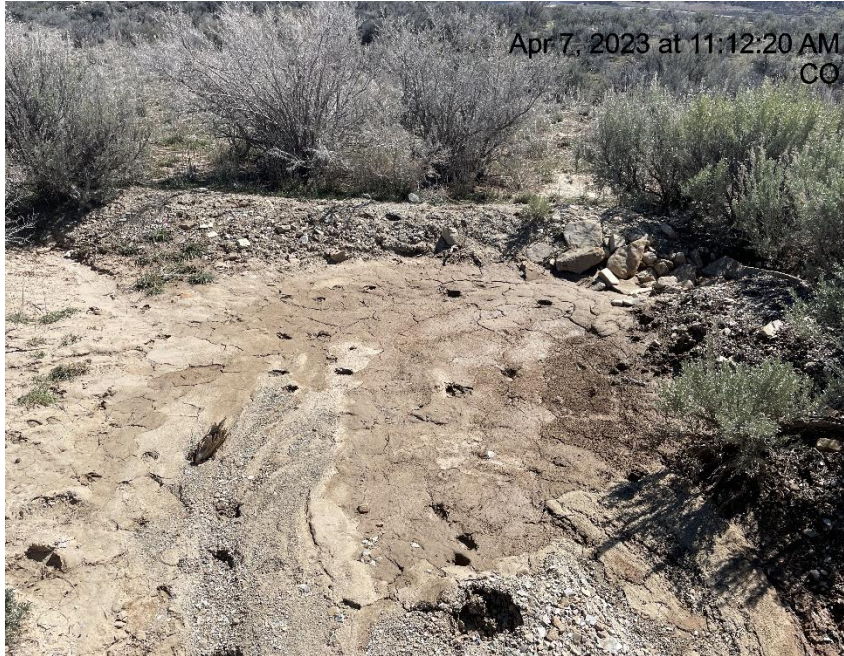
Photo # 4608 Sediment trap needs maintenance
