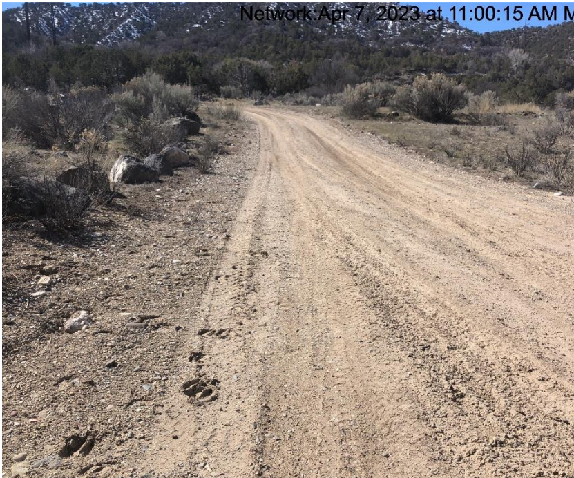
Photo #9565 Insufficient tracking BMP at entrance to location.
