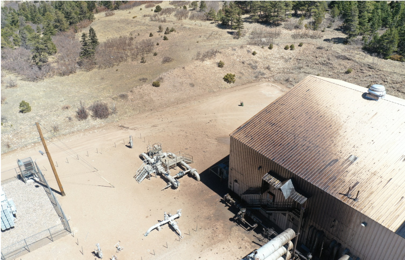
Photo 1. Drone aerial photo facing northeast at the Drill site 3 compressor. There was a leak that has blackened the facility and areas of the ground and sprayed out to the northeast off the location.
