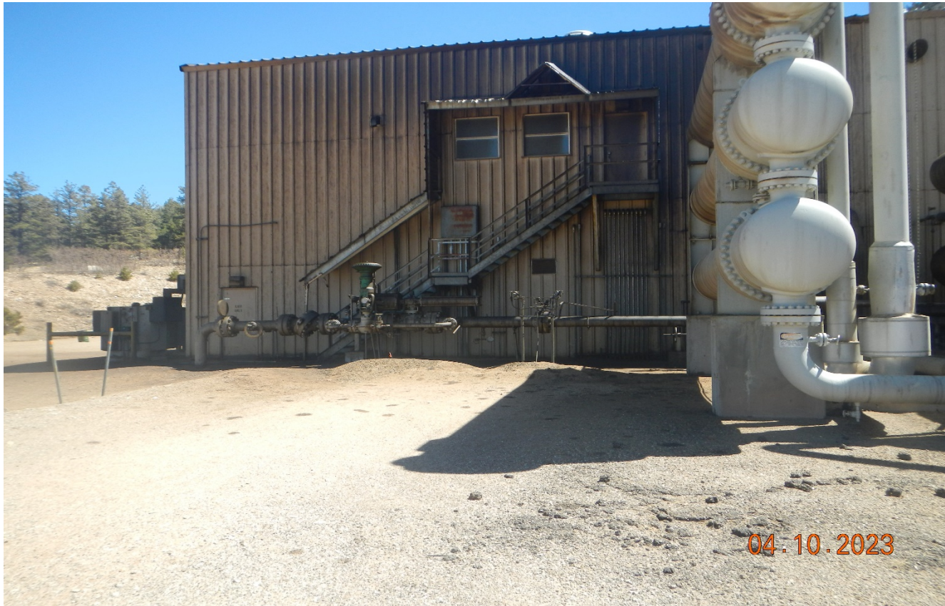
Photo 3. Facing east at the Drill site 3 compressor. There was a leak that has blackened the facility and areas of the ground that needs to be cleaned up.
