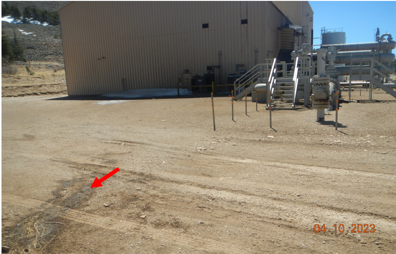
Photo 5. Facing southeast at the north side of the Drill site 3 compressor. There is oil stained soils that have sprayed out north of the compressor.
