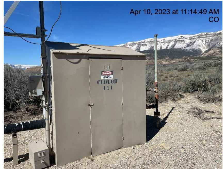
Photo # 4862 Meter calibration info not conspicuously posted
