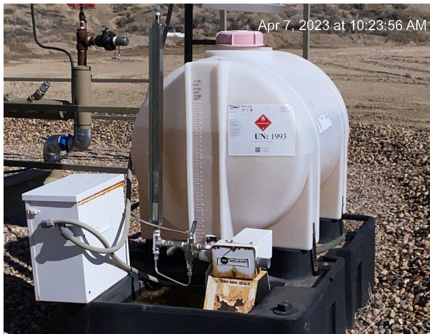
Labeling added to chemical tank
