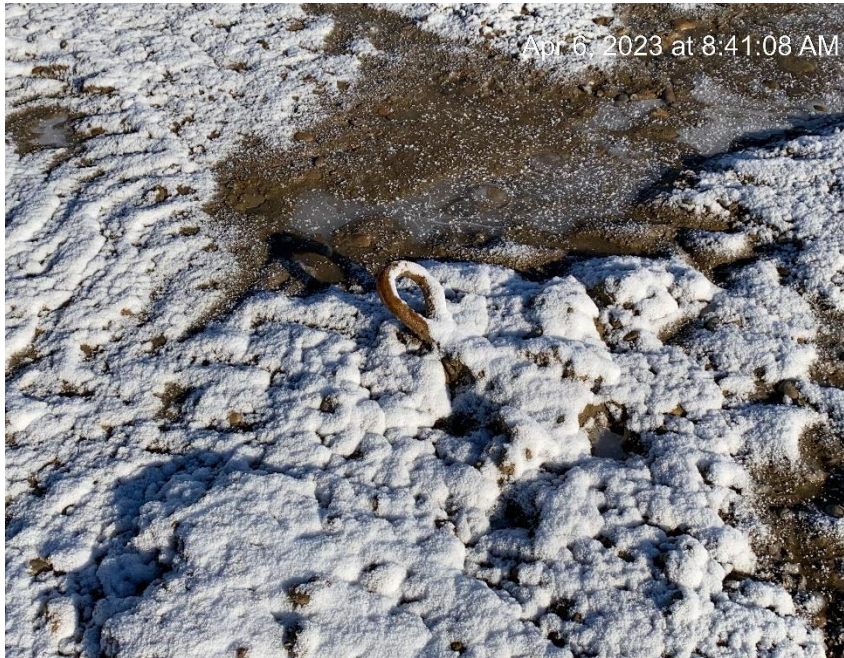
Unmarked anchor on SE corner
