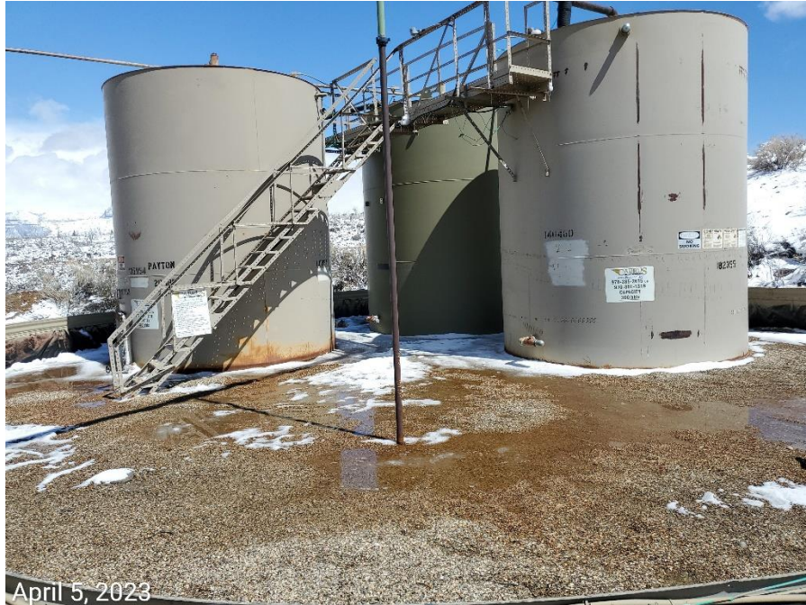
Photo 4: Secondary containment at the three 300 bbl produced water/condensate tanks is inadequate to contain a spill.
