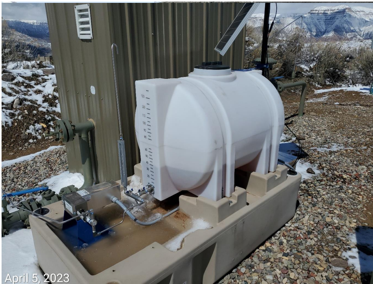
Photo 6: Chemical container lacks required marking/labeling/signage.
