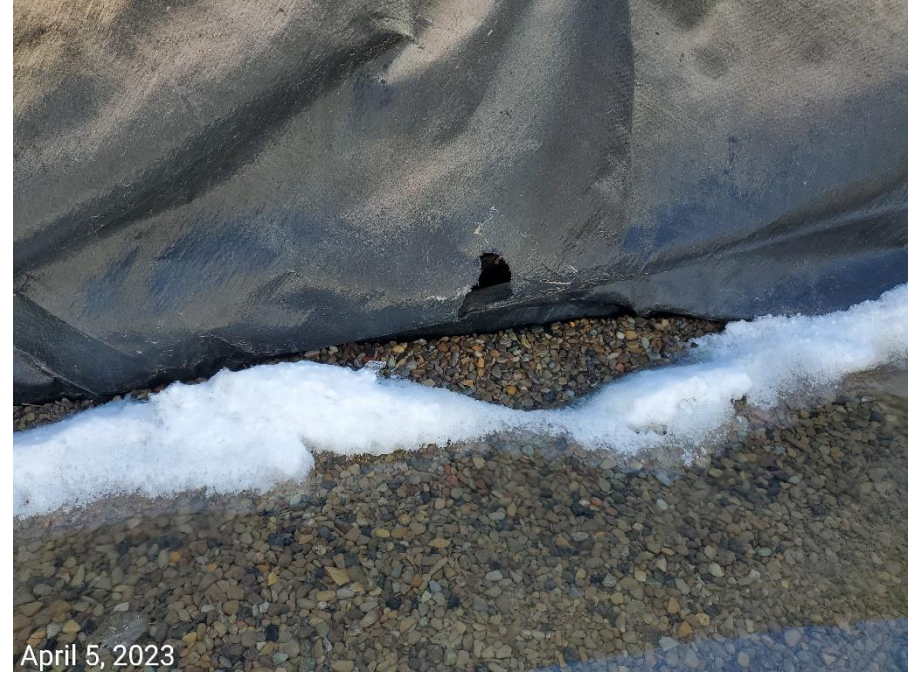
Photo 4: Secondary containment at the three 300 bbl produced water/condensate tanks is inadequate to contain a spill.
