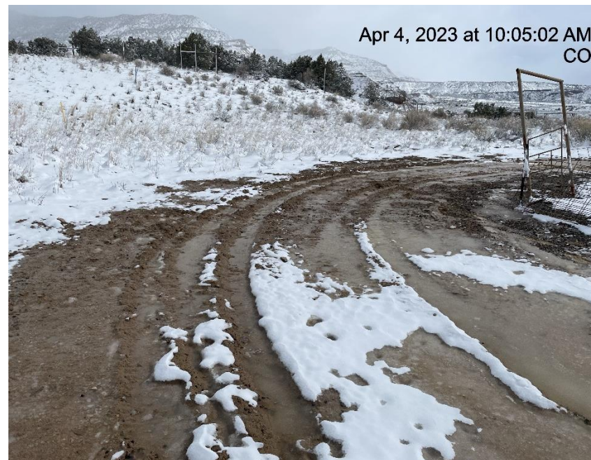
Photo # 4117 Lack of stabilization/Insufficient tracking BMP's
