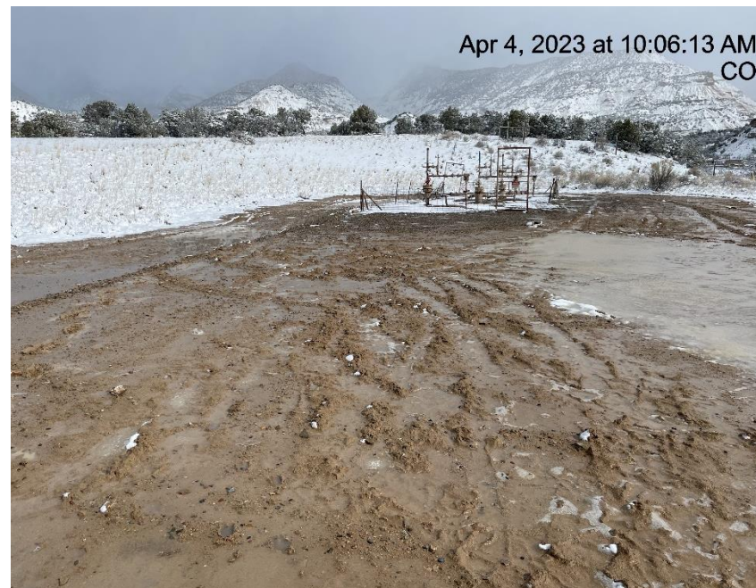
Photo # 4172 Lack of stabilization/Insufficient tracking BMP's
