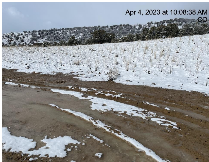
Photo # 4178 Lack of stabilization/Insufficient tracking BMP's
