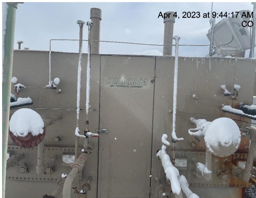
Photo # 4147 Meter calibration info not conspicuously posted
