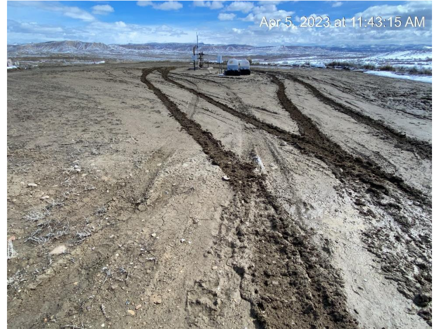
Lack of stabilization at entrance to location
