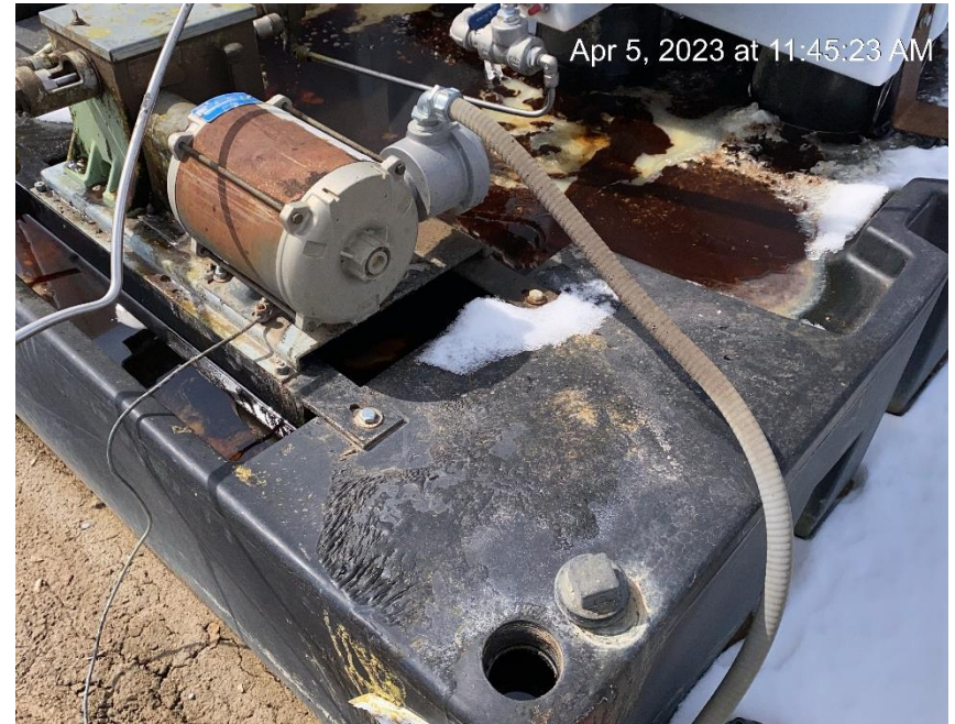
Chemical containment full in need of maintenance
