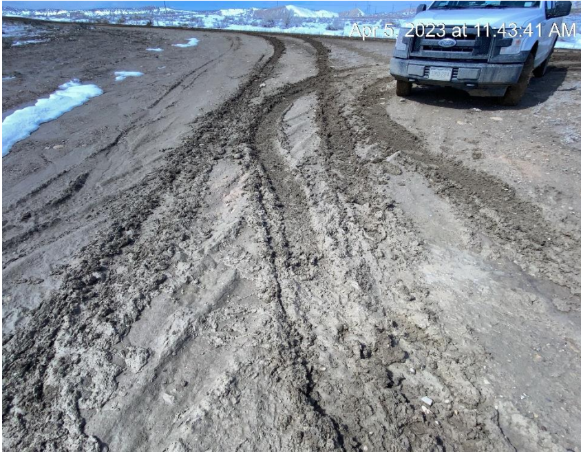
Vehicle tracking on to access and lease roads.
