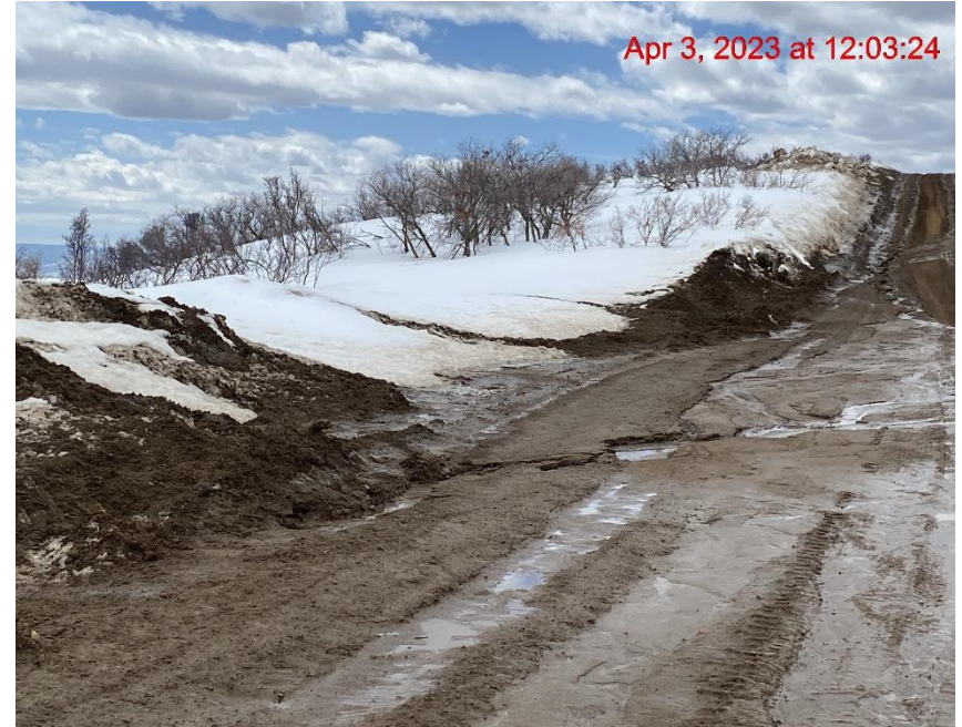
Lease Road Degradation/Transport of Sediment – Photo #01829
