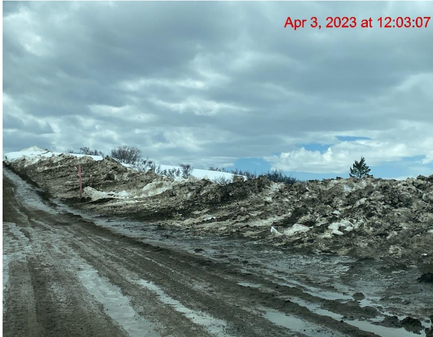
Lease Road Degradation/Transport of Sediment – Photo #01828
