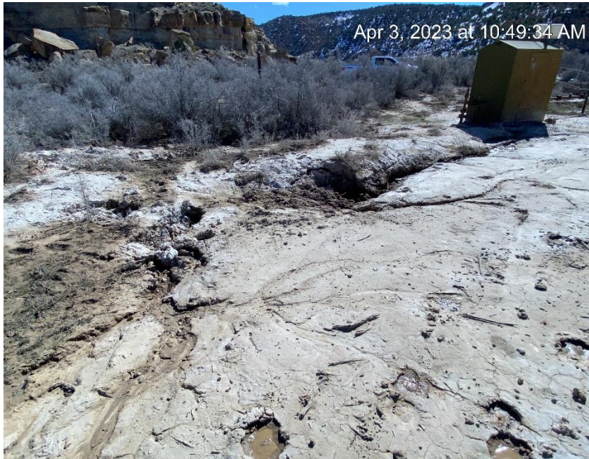
Erosion between separator and meter house draining into Douglas Creek
