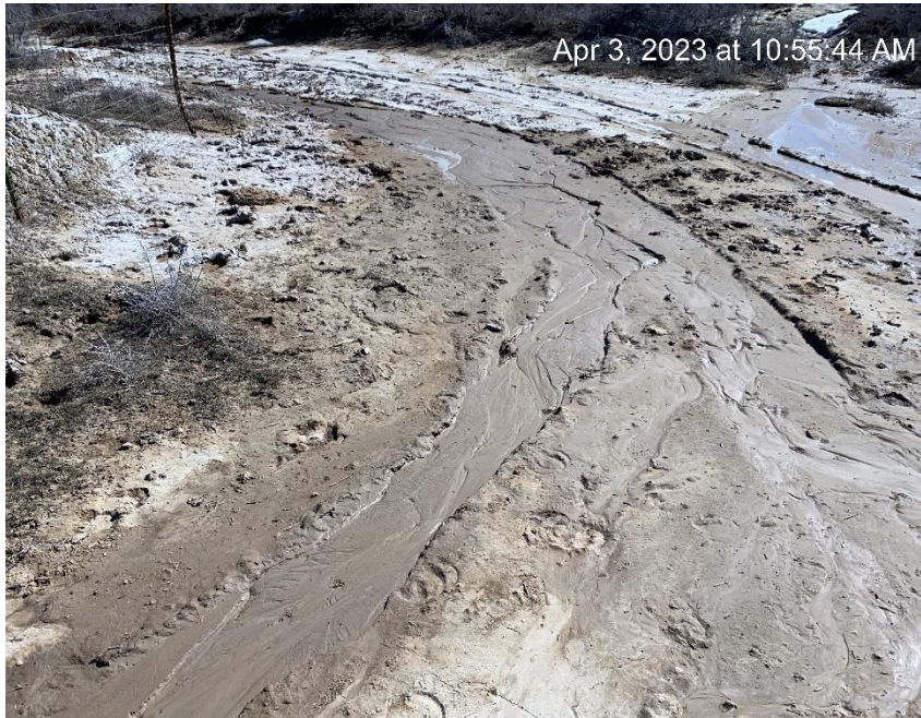
Stormwater and sediment migration on to lease road and location
