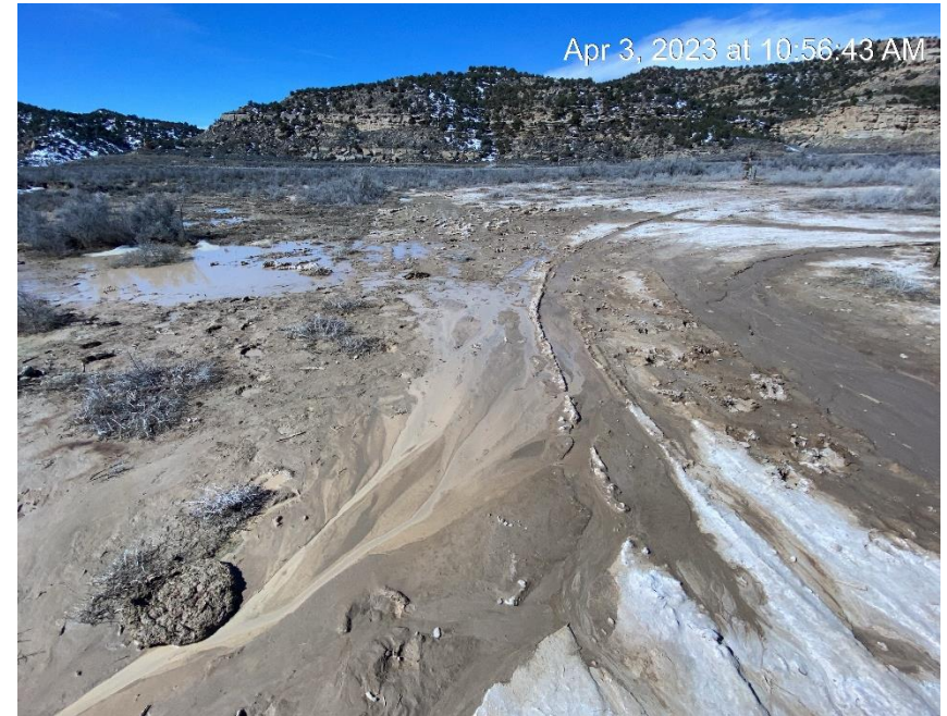
Stormwater and sediment migration on to lease road and location
