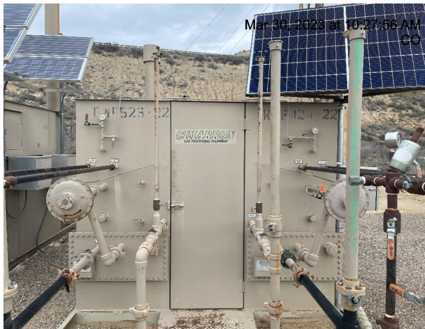
Photo # 3632 Meter calibration info not conspicuously posted
