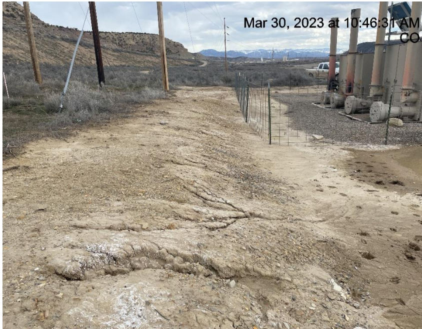
Photo # 3662 Rill erosion & transport of sediment onto location
