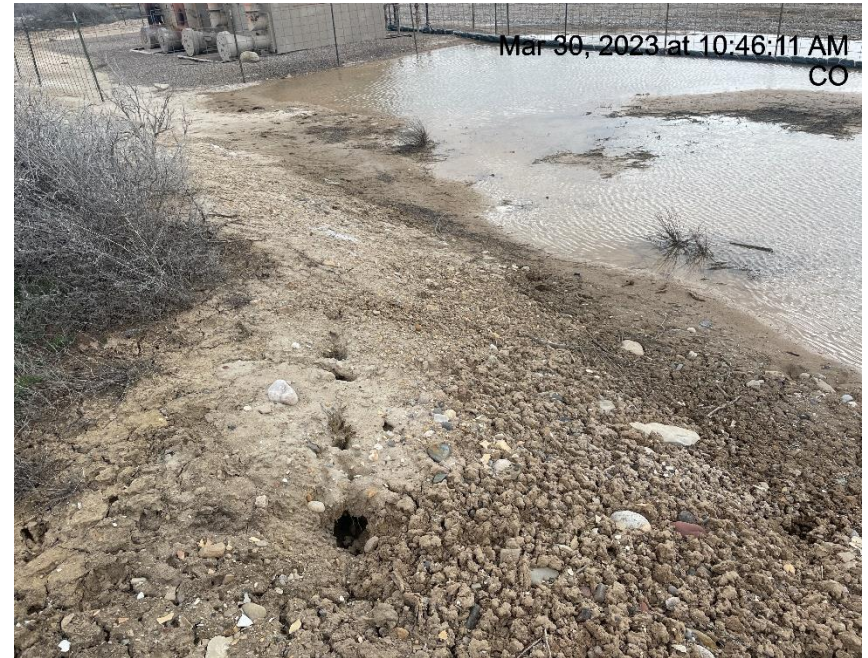
Photo # 3660 Tunnel erosion
