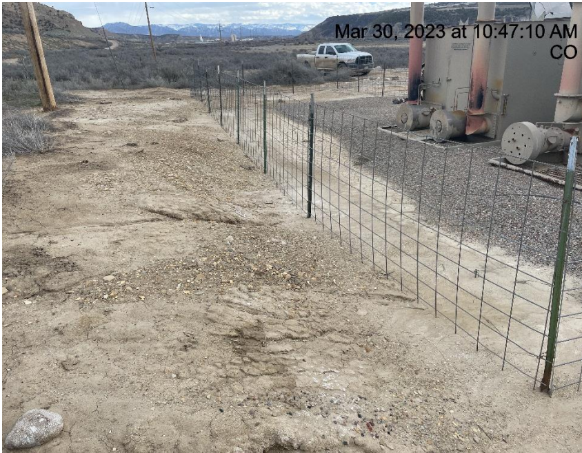
Photo # 3664 Rill erosion & transport of sediment onto location
