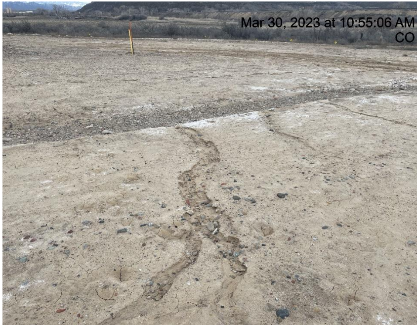
Photo # 3688 Rill erosion (SW side of pad)
