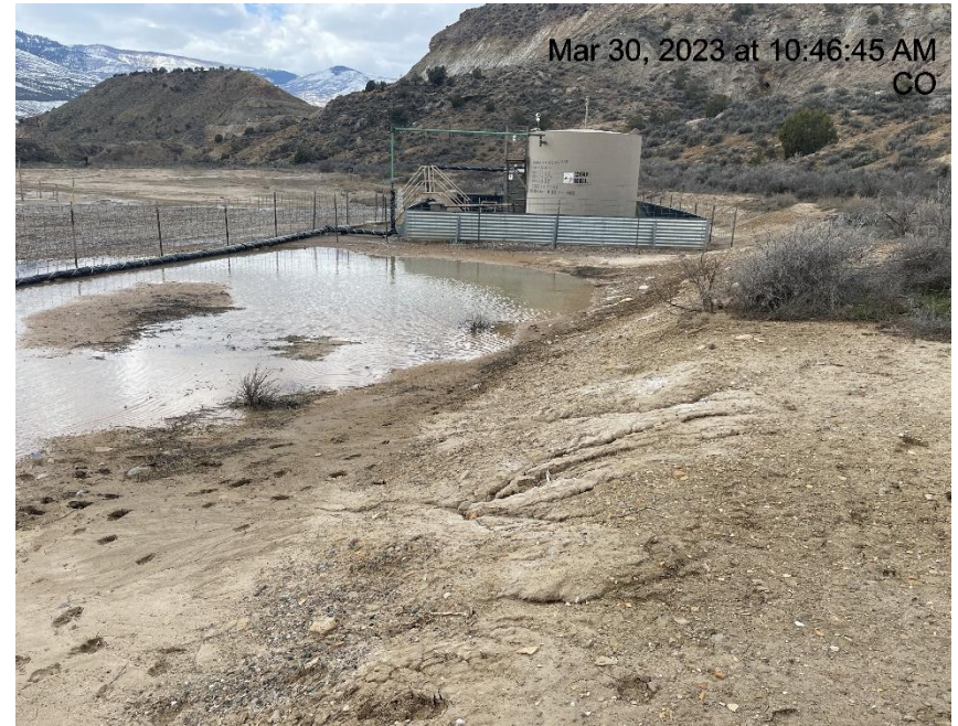
Photo # 3663 Rill erosion & transport of sediment onto location
