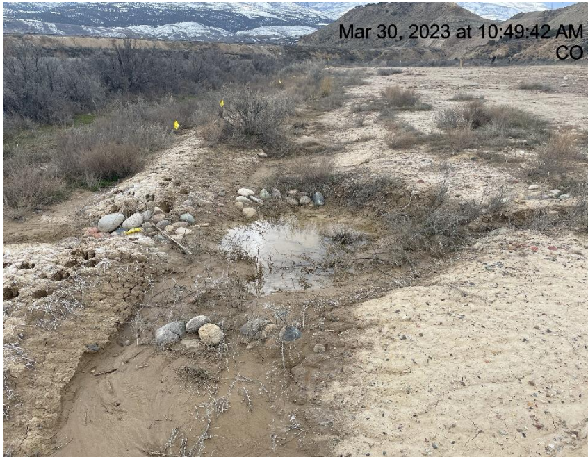
Photo # 3671 Sediment trap needs maintenance (SE corner of pad)
