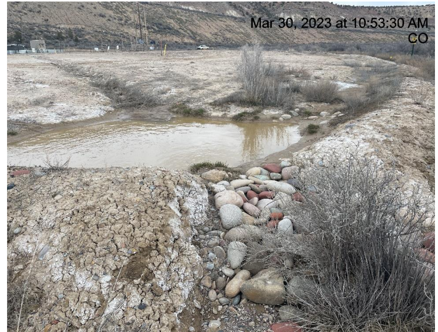
Photo # 3684 Sediment Trap needs maintenance (SW side of pad)
