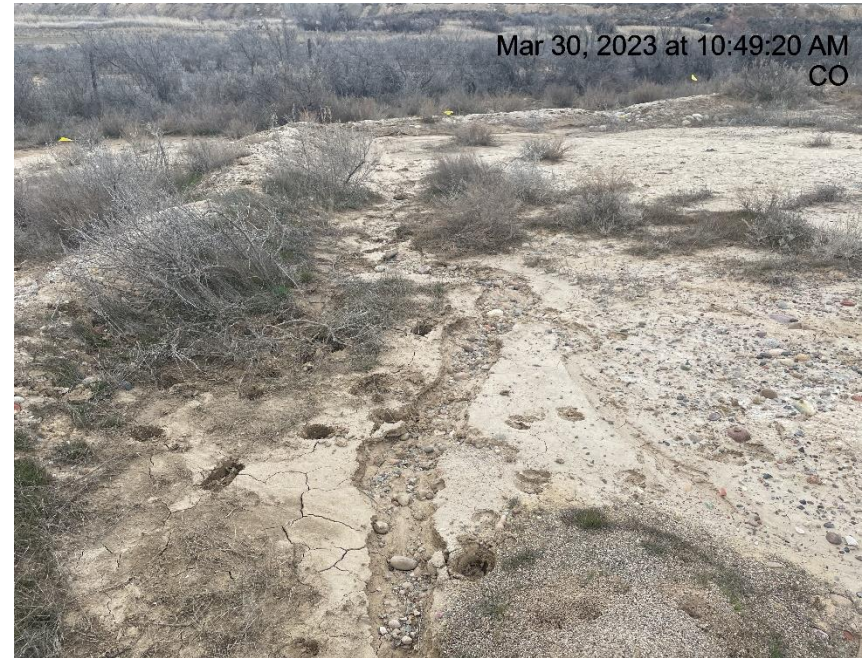
Photo # 3669 Rill erosion (SE side of pad)
