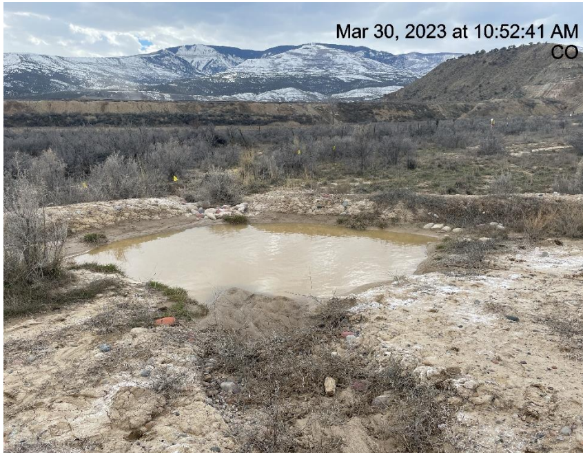
Photo # 3681 Sediment Trap needs maintenance (SW side of pad)
