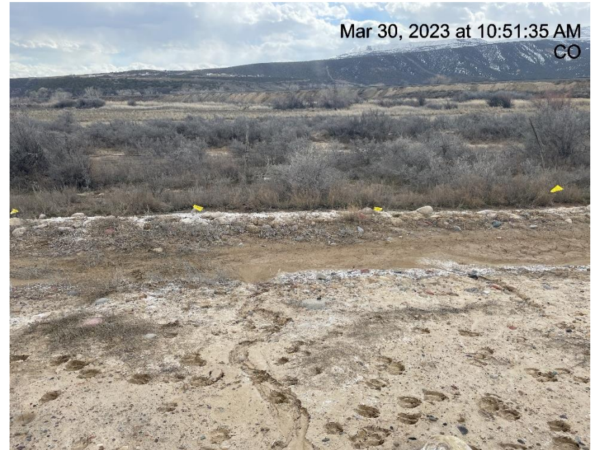
Photo # 3675 Rill erosion (south side of pad)
