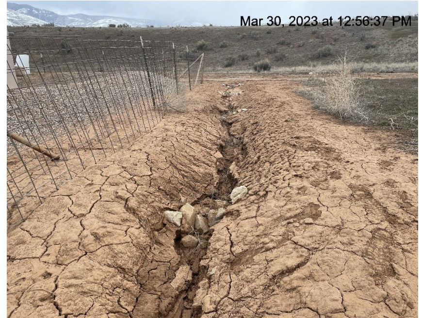
Photo # 3837 Ditch & check dams need maintenance
