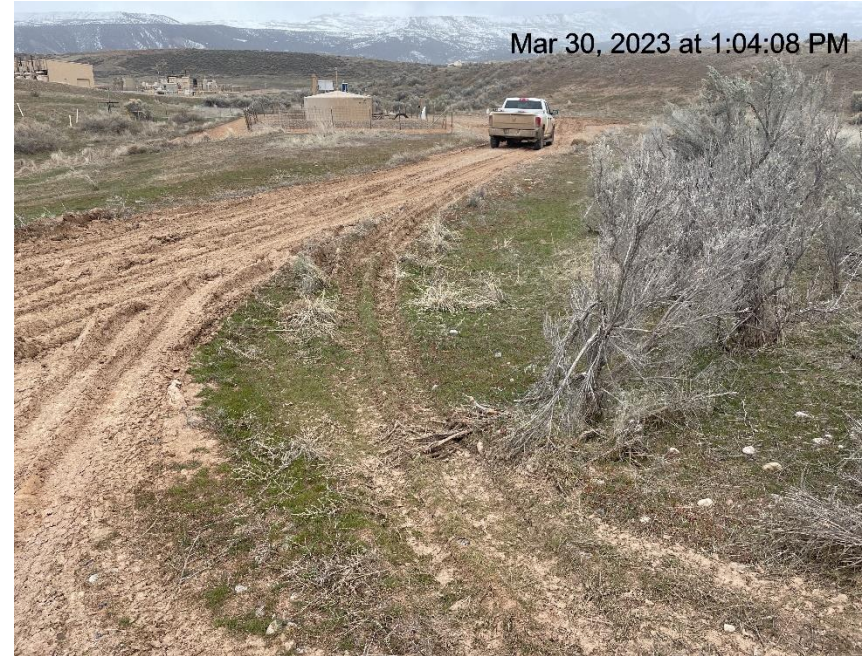
Photo # 3854 Failure to minimize surface disturbances and restrict vehicle traffic to designated access road
