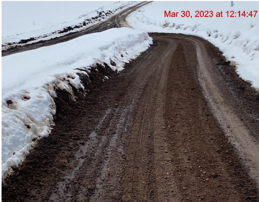
Lease Road Degradation/Transport of Sediment – Photo #01754
