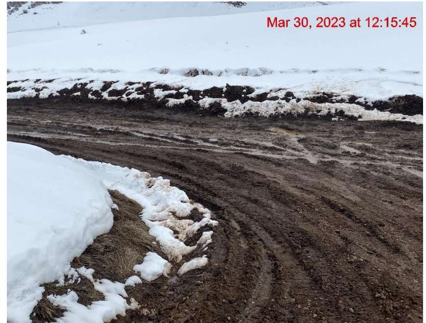
Lease Road Degradation/Transport of Sediment – Photo #01756
