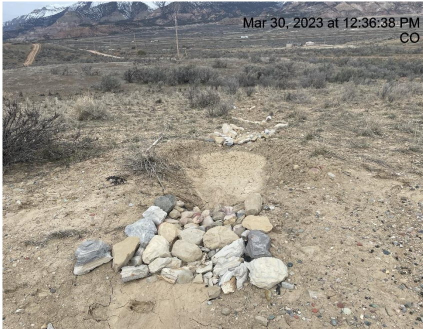
Photo # 3798 Sediment Trap needs maintenance (upper tier of pad, NW edge of pad across from wellheads.)
