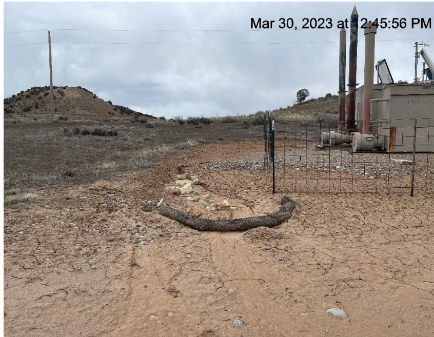
Photo # 3814 Erosion/transport of sediment off location/insufficient BMP's
