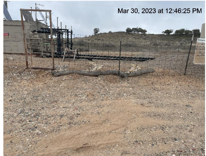
Photo # 3816 Erosion/transport of sediment off location onto lease road/insufficient run off controls/BMP's
