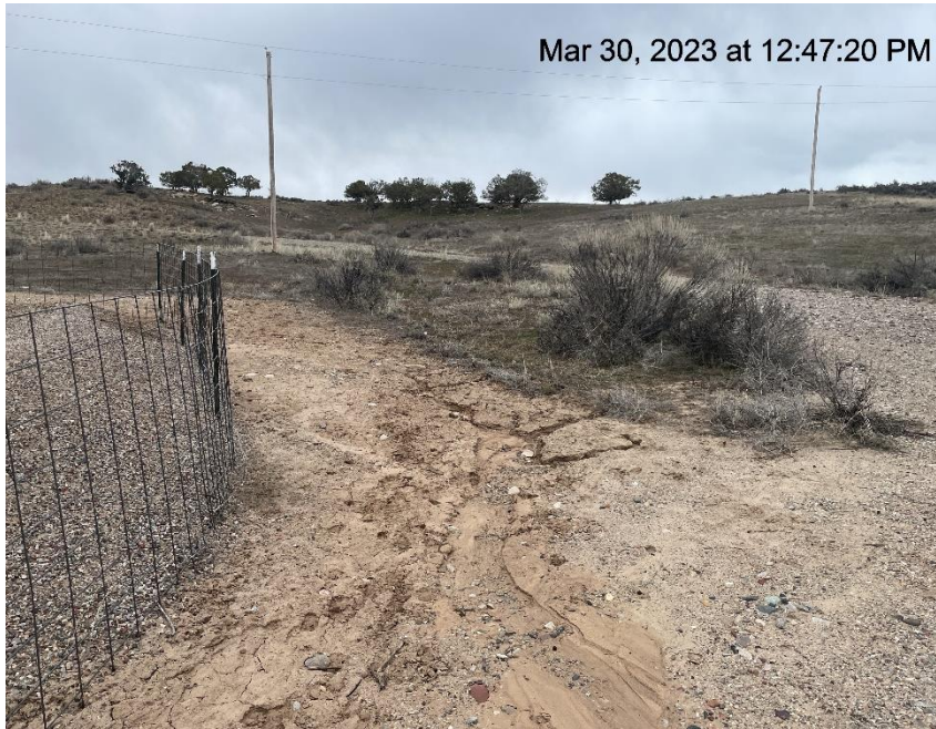
Photo # 3820 Rill erosion & transport of sediment off location onto lease road/insufficient BMP's
