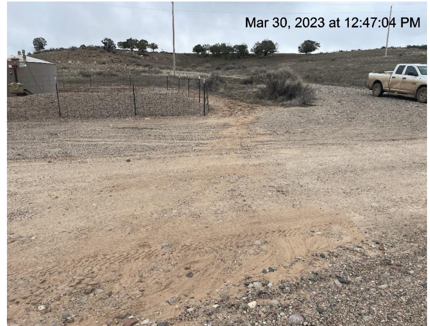
Photo # 3818 Rill erosion & transport of sediment off location onto lease road/insufficient BMP's
