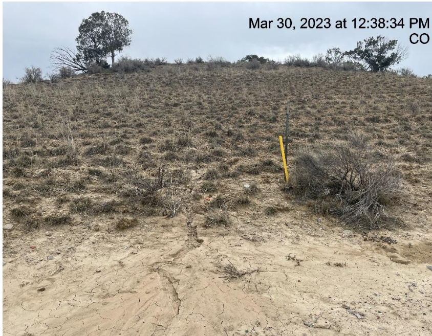
Photo # 3803 Rill erosion & transport of sediment onto location (upper tier NE side of pad)
