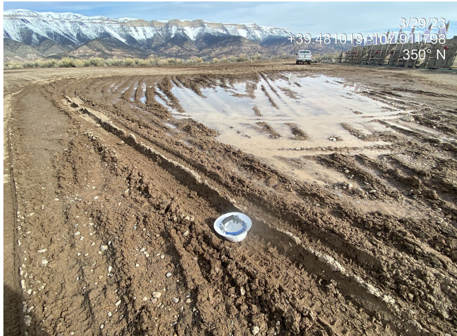
Photo 2. Photos show a lack of stabilization of the working pad surface.
