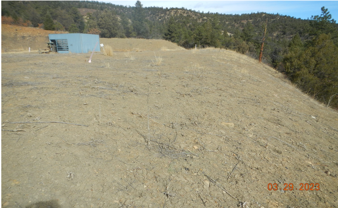
Photo 3. Facing toward the fill slope which needs to be reseeded and stabilized. There are also noxious weeds in this area (Canada thistle) which will need to be controlled.
