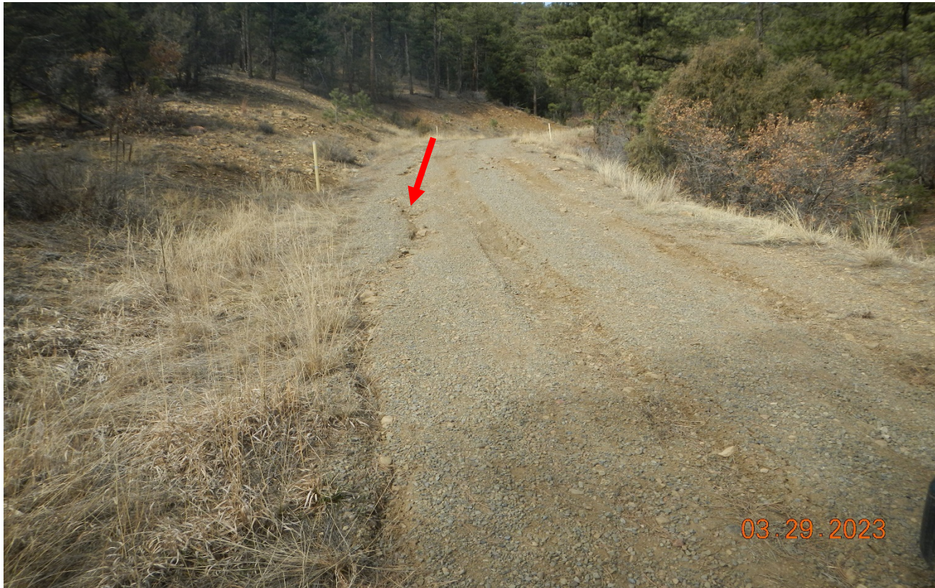
Photo 1. Facing toward the access road. There are signs of erosion from stormwater not diverted toward the culvert. Grading should be performed to direct stormwater toward the culvert.
