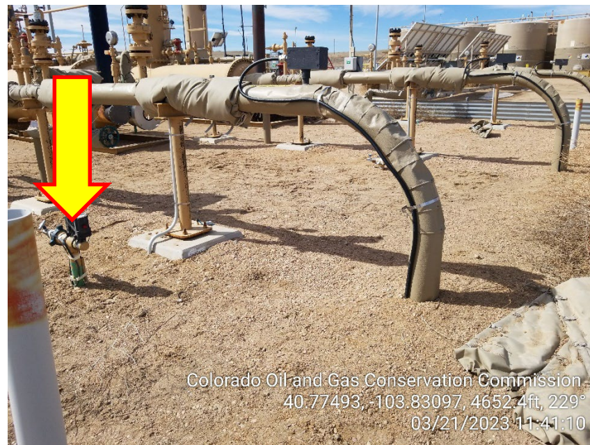
Photo 14 – Unmarked Risers
