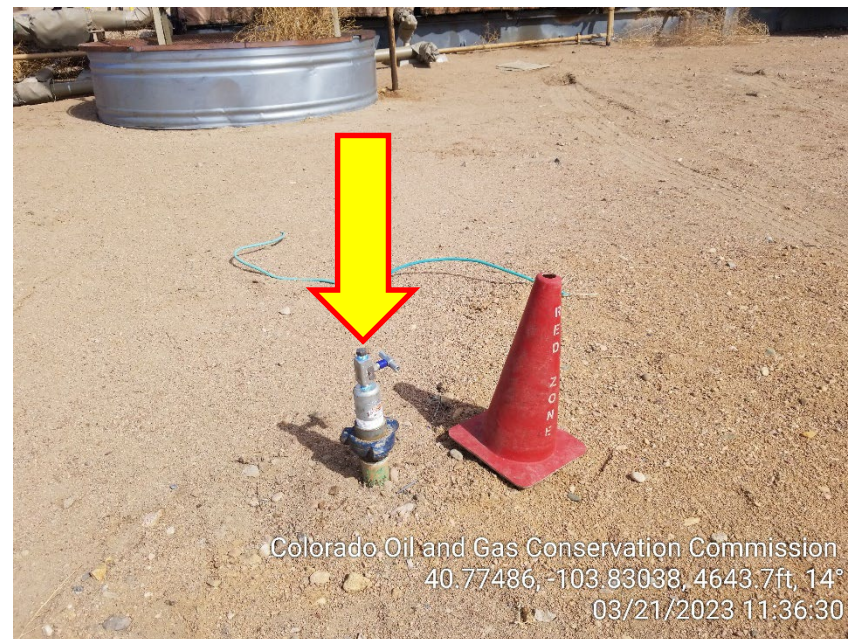
Photo 8 – Unmarked Riser
