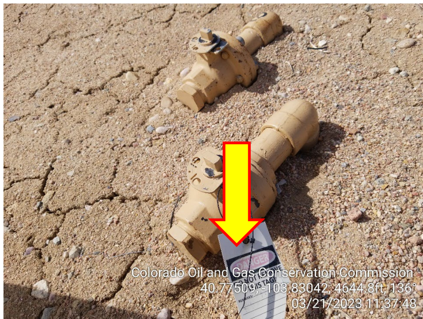
Photo 9 – Unmarked Riser – Tag Faded
