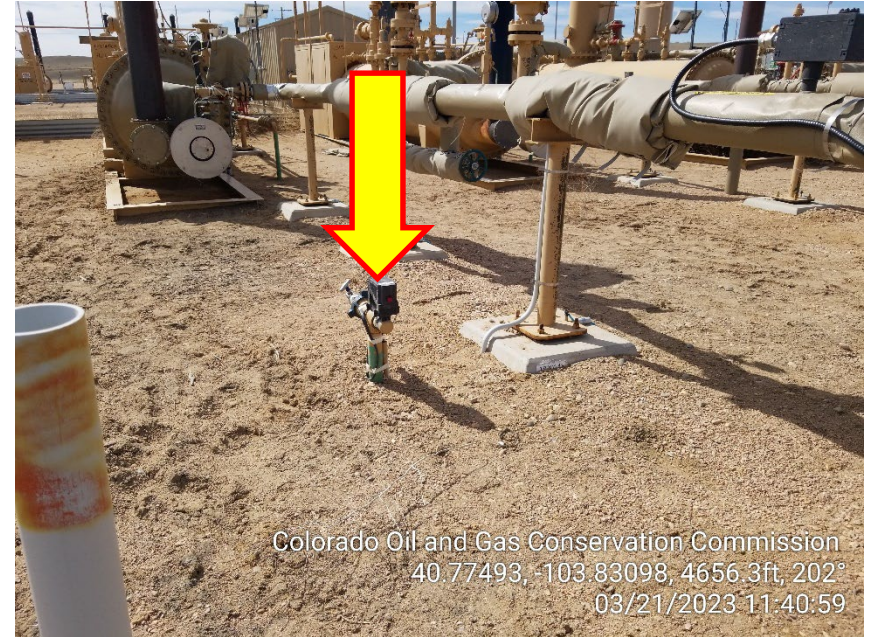
Photo 12 – Unmarked Riser
