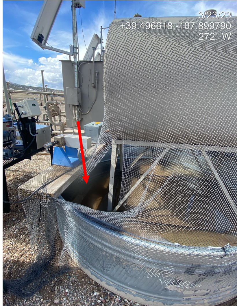
Photo 3. Photo shows a wildlife protection BMP in disrepair.
