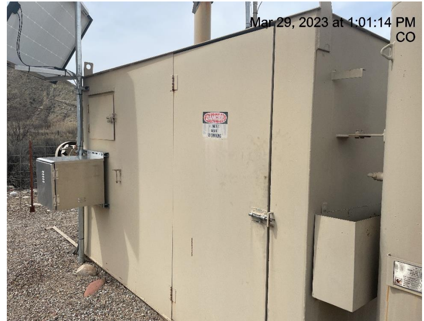
Photo # 3592 Meter calibration info not conspicuously posted
