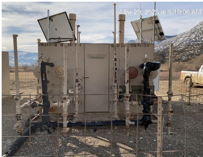
Gas meter calibration card not conspicuously posted.
