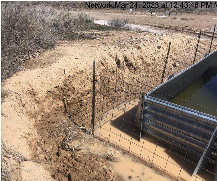
Photo #9406 Run on to location is not being controlled.
