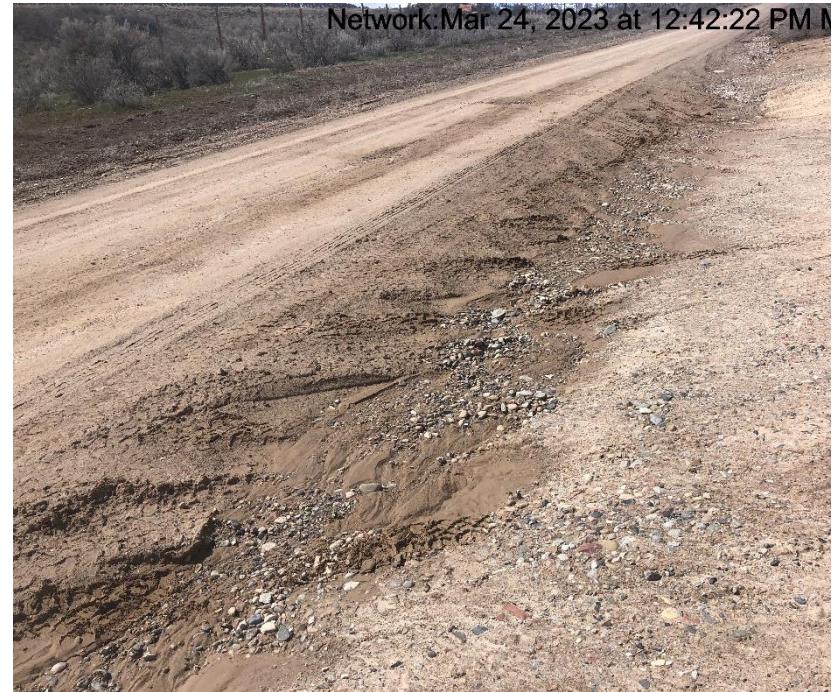
Photo #9396 Insufficient tracking BMP at entrance to location.
