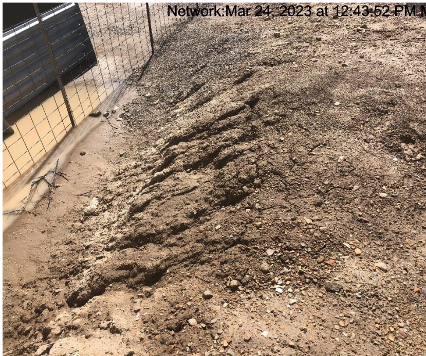
Photo #9403 Rill erosion on berms.
