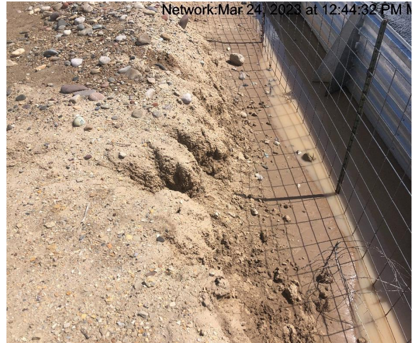
Photo #9407 Run to location is not being controlled.
