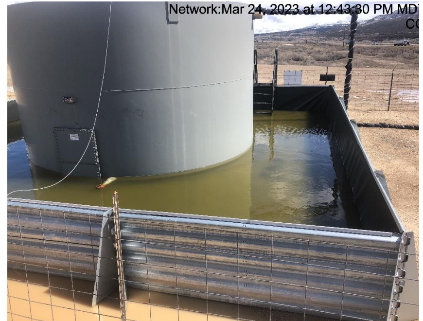
Photo #9400 Capacity reduced due to Stormwater in tank containment
