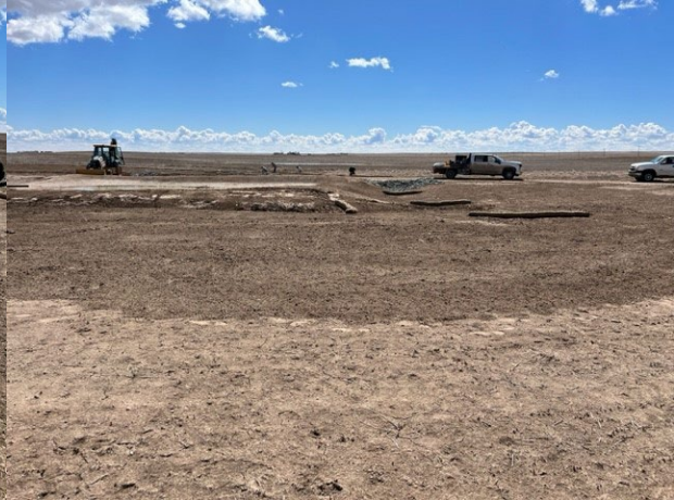
View from north of the west most pit. sediment migration mitigated, Areas of disturbance scarified and seeded. Waddles placed up stream of the armored sediment trap.
