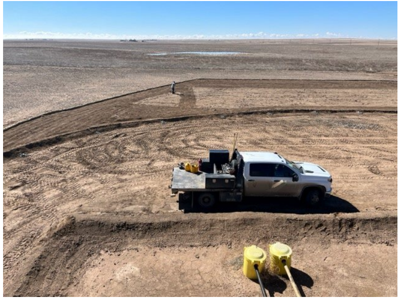
Check dams installed at current working surface berm and ditch. Berm has been compacted by equipment and then walked and recompactd by personnel.
