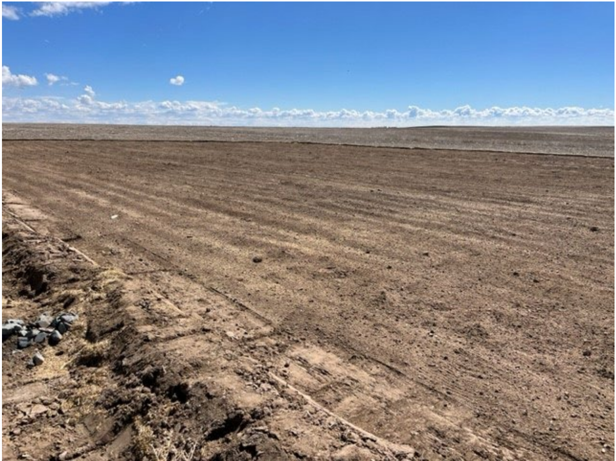
Prior working surface for the April well and pump jack. Scarified and seeded.
