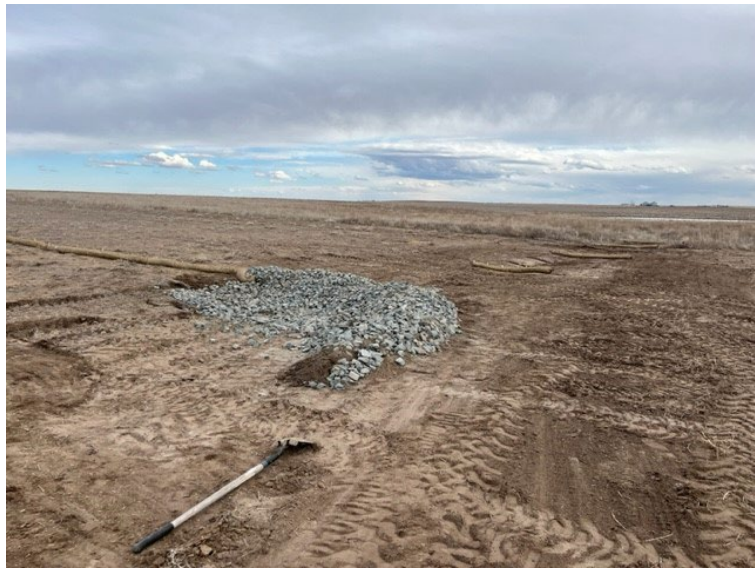
Farthest south sediment armored sediment trap. Series of waddles below.
