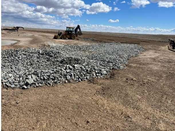
Pad entrance water bar and up stream sediment trap.
