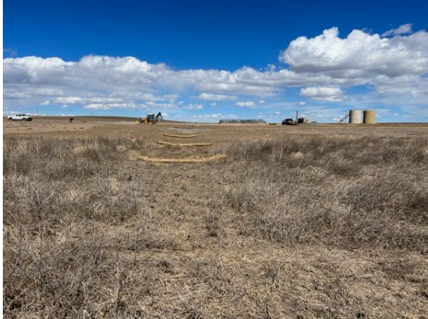
South of the location looking north. Sediment migration mitigated; waddles installed below the lower armored sediment trap. All working and reclaimed areas scarified and seeded.
