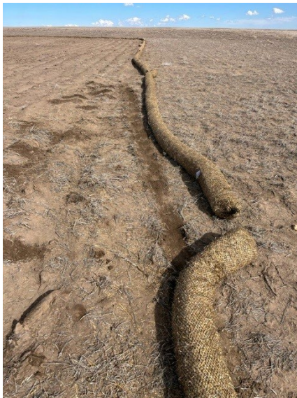
Waddles keyed slightly prior to staking to ensure full contact with the ground.
