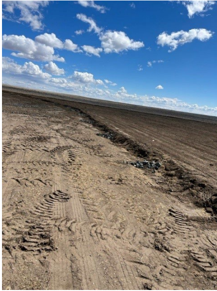
Check dams installed at current working surface berm and ditch. Berm has been compacted by equipment and then walked and recompactd by personnel.
