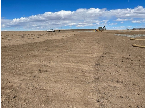
Area west of the April reclaimed working surface scarified and seeded.
