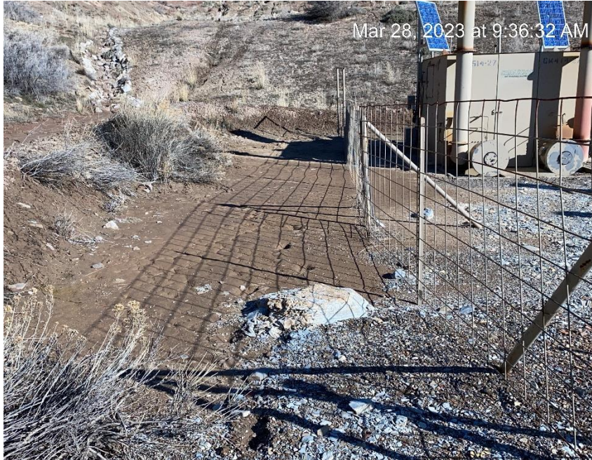
Sediment migration on separator pad
