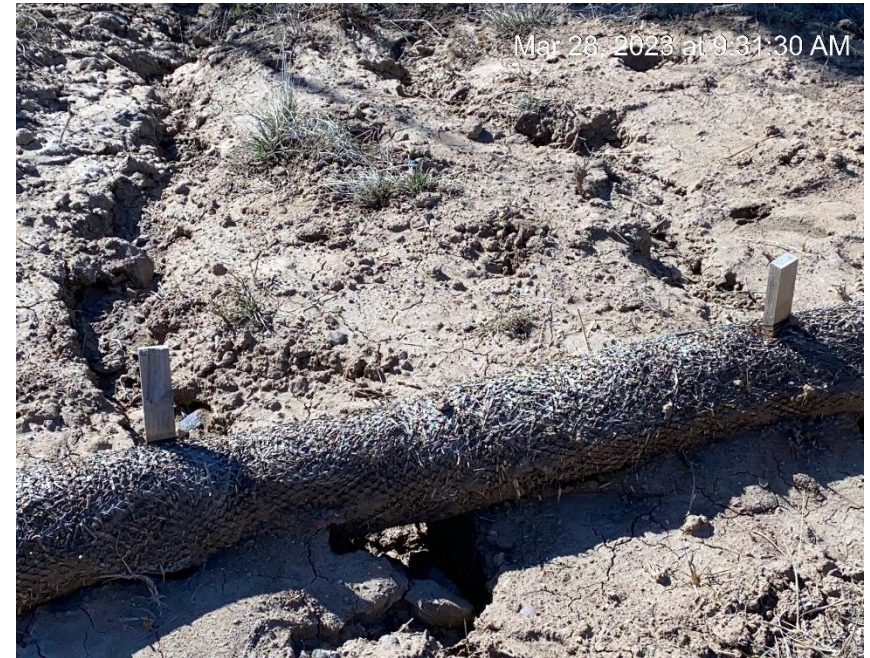
Erosion underneath wattle
