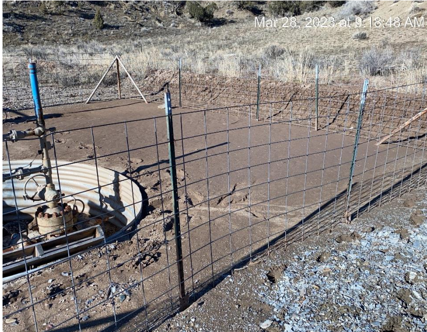
Sediment migration around wellheads
