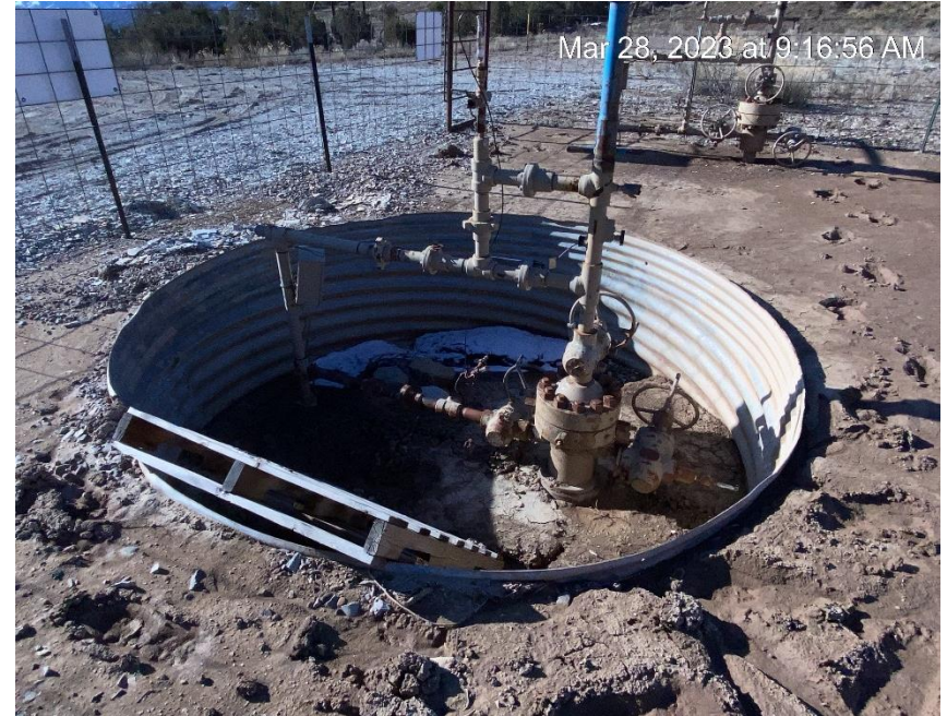
Open cellar around GM 224-34 wellhead
