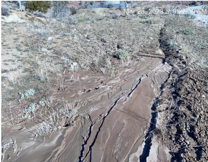
Erosion and sediment migration from tank battery and upper well pad.
