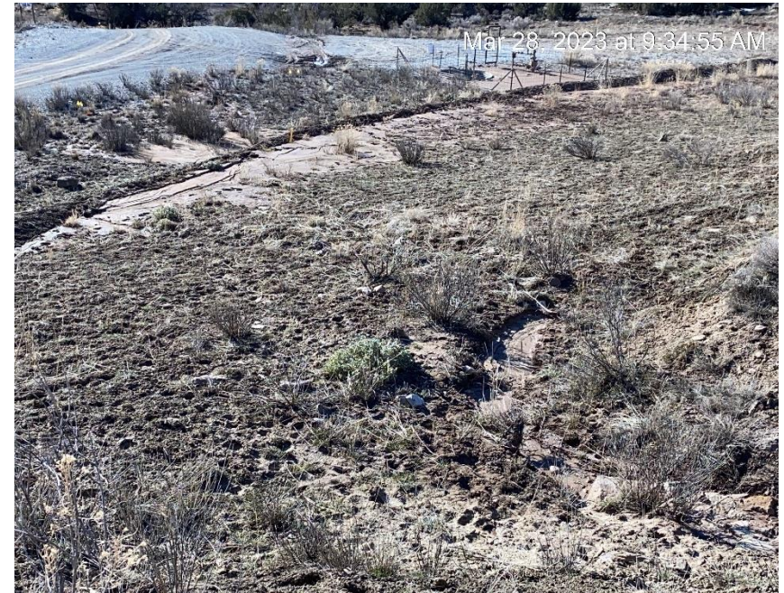
View from tank battery. Erosion. Sediment migration across location.
