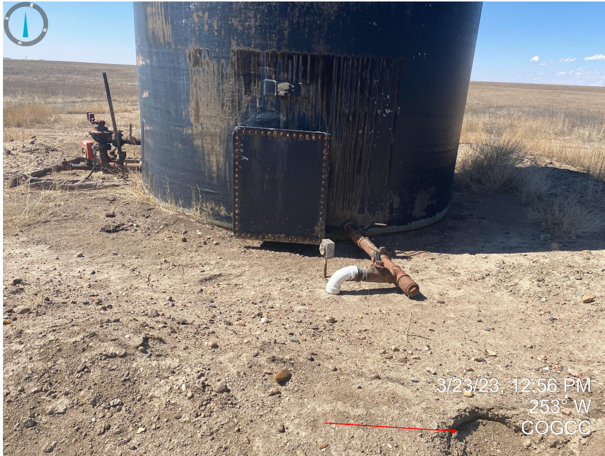
Photo 7. Facing west at battery. Earthen berm appears inadequate to contain 150% of tank volume with evidence of animal burrows, breached berm walls, and inadequate free board.
