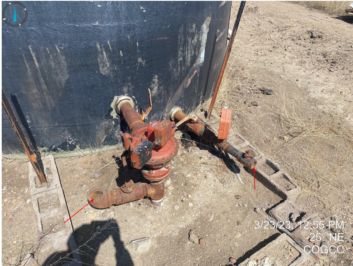
Photo 6. Loadout lines without bull plugs or caps.
