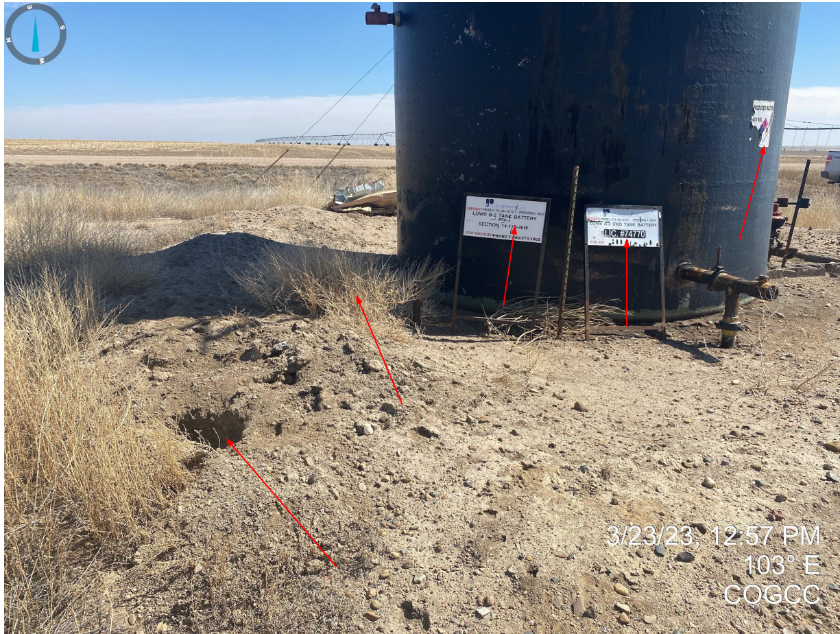
Photo 9. Facing east at battery. Animal burrow within earthen berm, undesirable vegetation (e.g. kochia) and illegible emergency contact/NFPA labels. Sign at left has two different emergency contact numbers.
