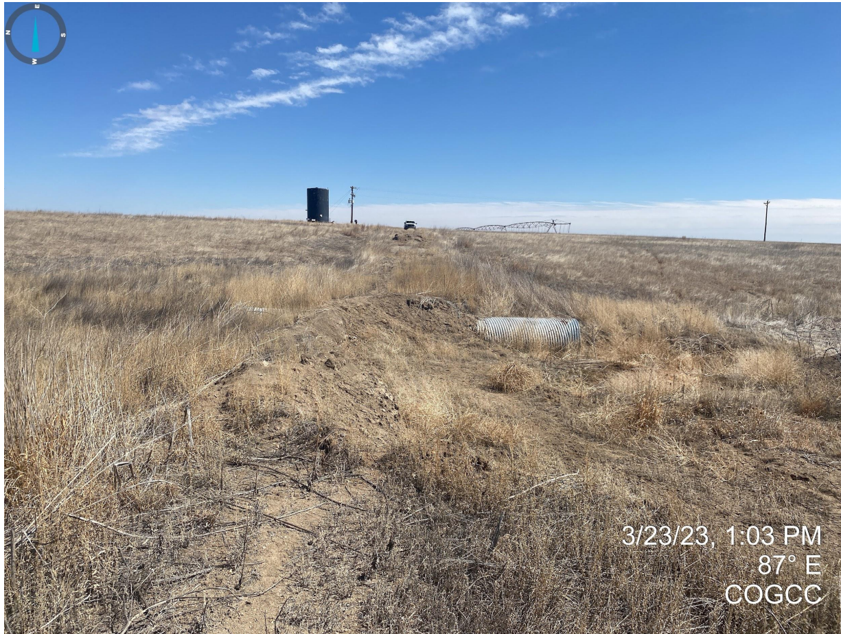
Photo 14. Facing east from access/lease road. It appears the road has been excavated and is not accessible to Staff or emergency services and will need to be repaired.
