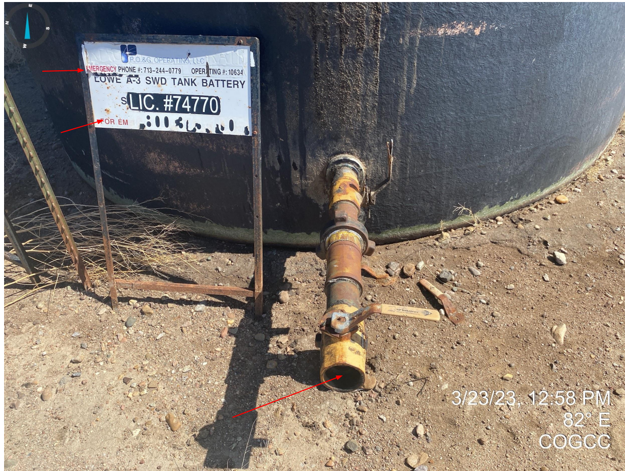
Photo 10. Loadout lines without bull plug/cap. See comments in Photo 9 for additional.
