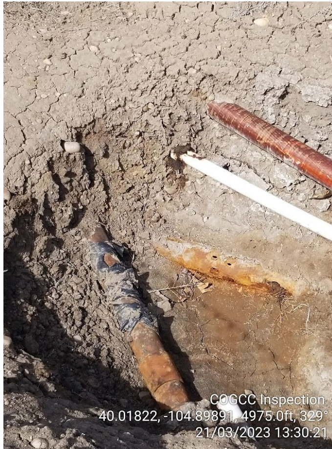
Photo 2 – Corroded pipes and staining at base of surface scraping.
