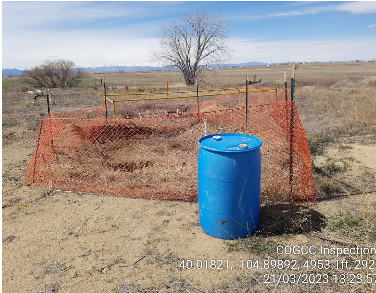
Photo 1 – Spill point. Surface scraping to expose pipelines, no remedial excavation
