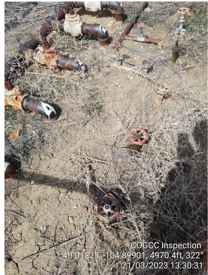
Photo 3 – Staining at header
