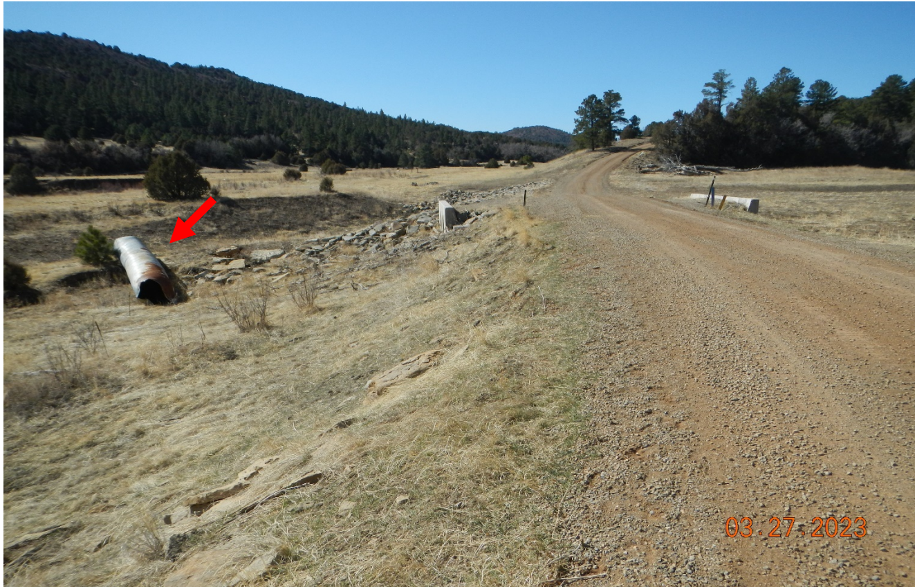
Photo 1. Facing southwest along the main road traveling to the location. The old culvert shown at red arrow needs to be removed.
