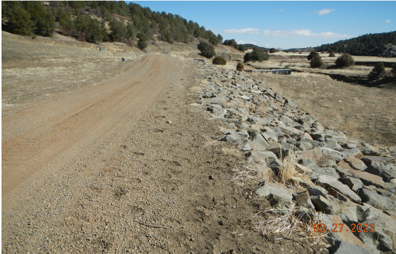
Photo 2. Facing back northeast along the road where repairs of the road were made including rip/rap for embankment stabilization.
